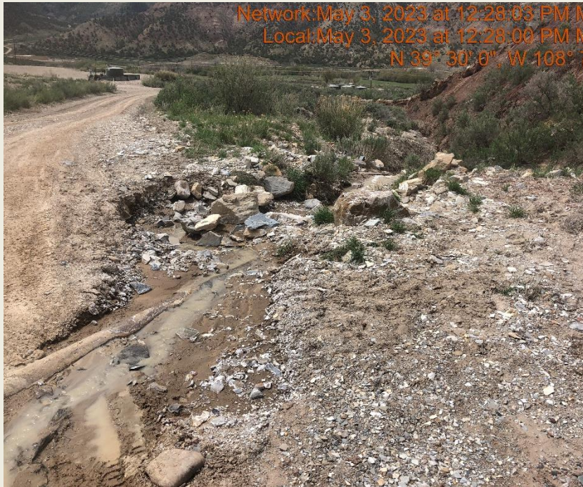
Photo #9864 -Culvert capacity insufficient.
