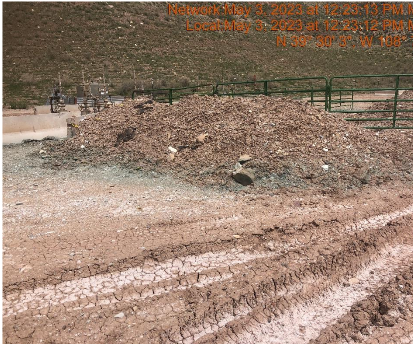
Photo #9853 Insufficient stock piled soils BMPs
