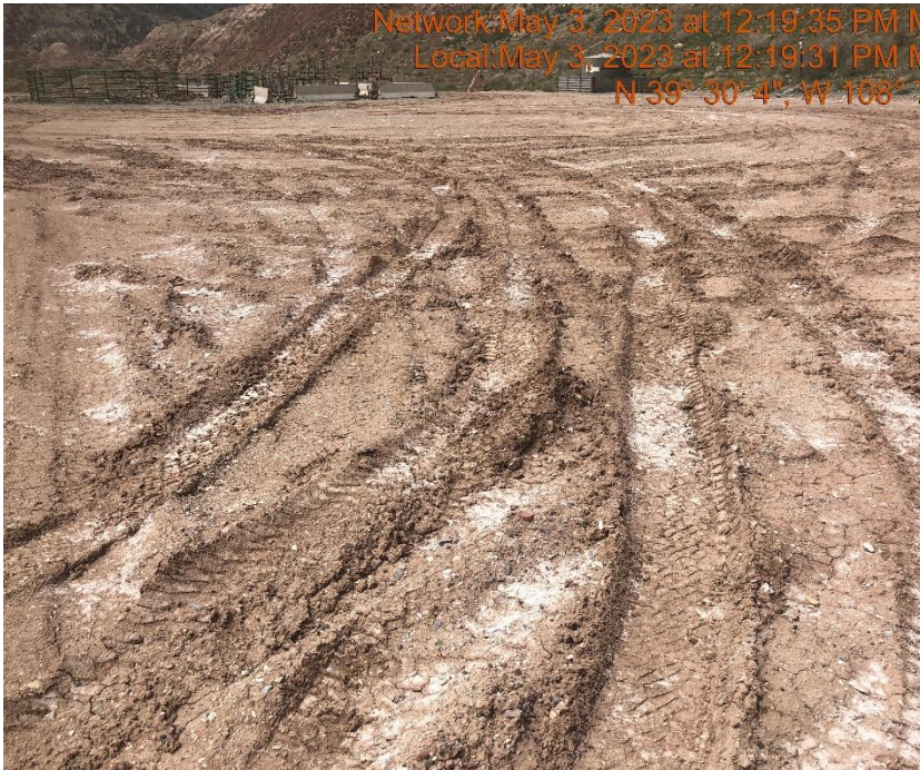
Photo #9840 Location lacks stabilization
