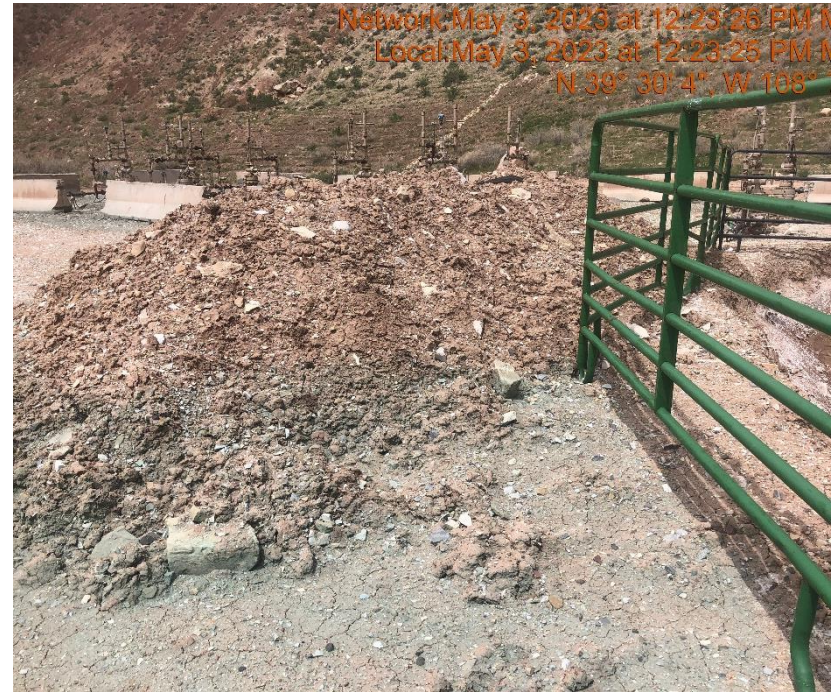
Photo #9854 Insufficient stock piled soils BMPs
