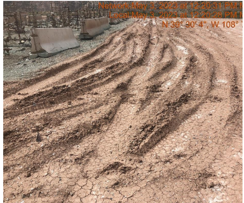
Photo #9844 Location lacks stabilization
