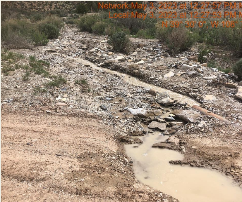
Photo #9862 Culvert capacity insufficient.
