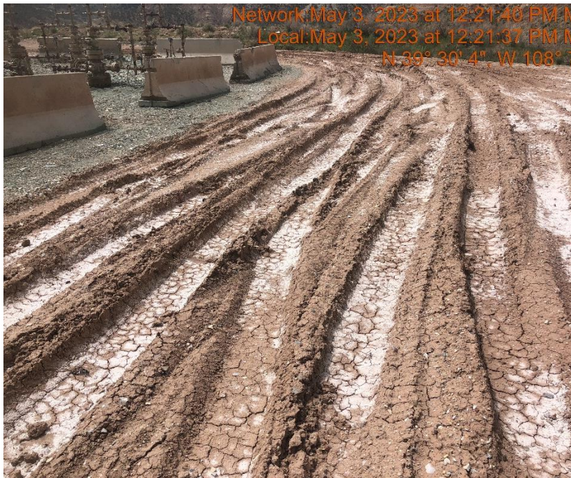
Photo #9848 Location lacks stabilization
