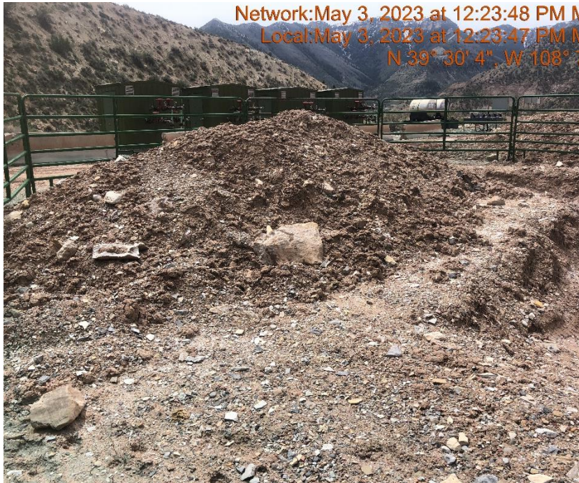
Photo #9855 Insufficient stockpiled soil BMPs
