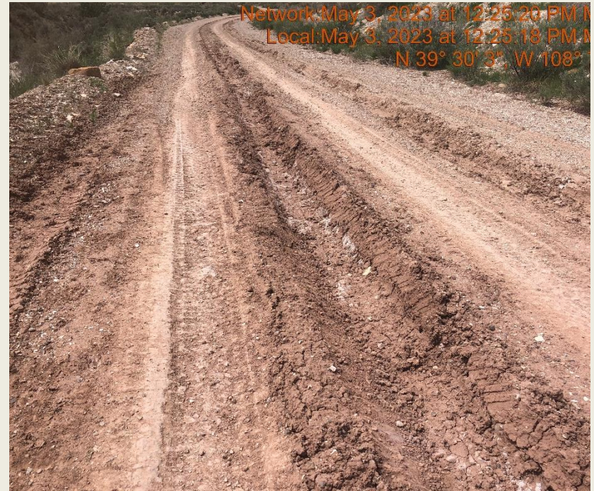
Photo #9860 Access road lacks stabilization
