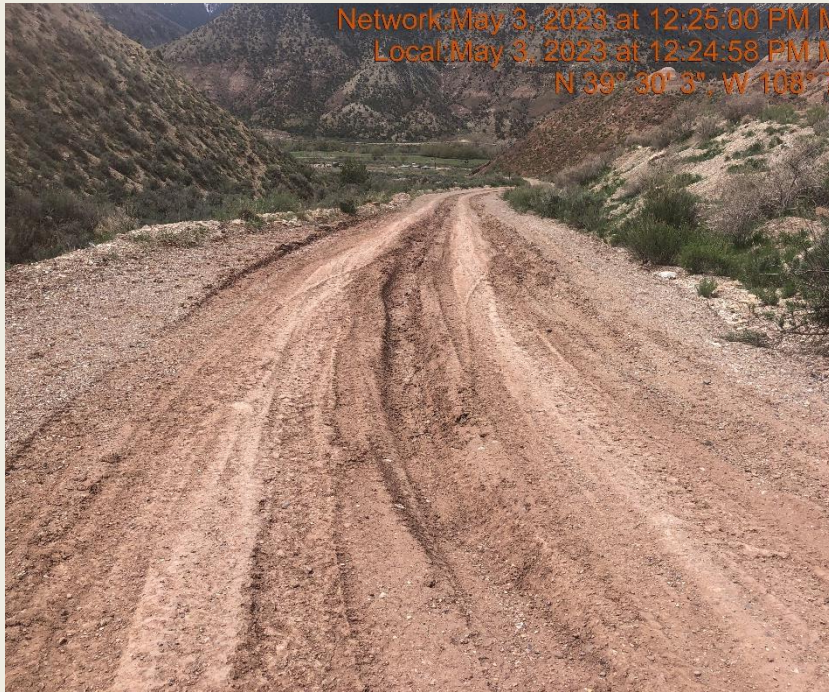
Photo #9859 Access road lacks stabilization
