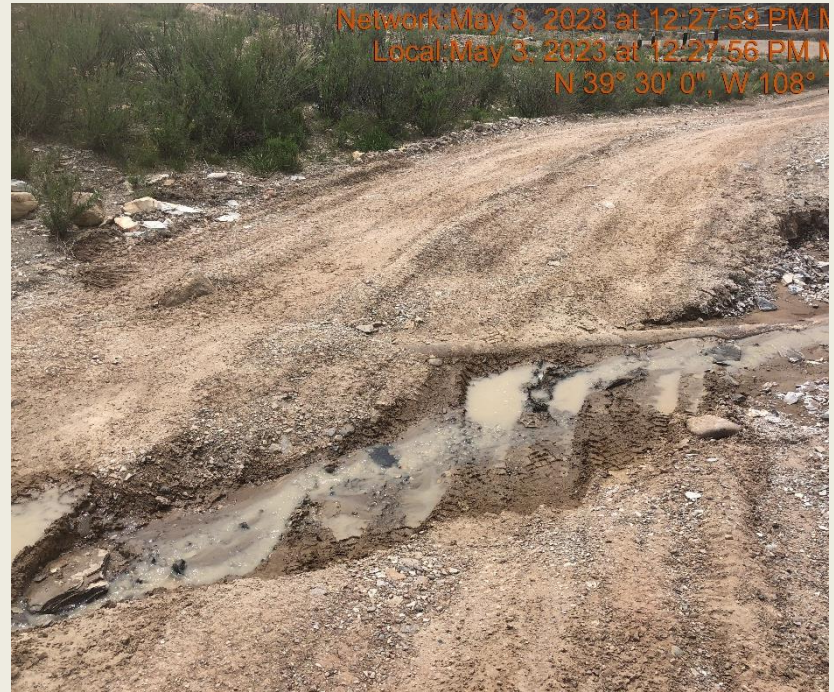
Photo #9863 Culvert capacity insufficient.
