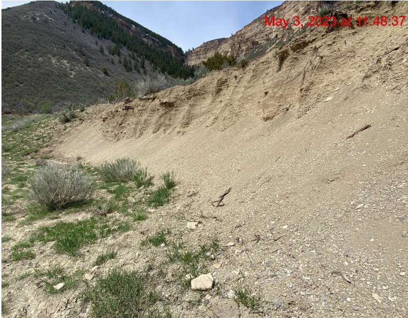
Cut Slope Eroding onto Location – Photo #02854
