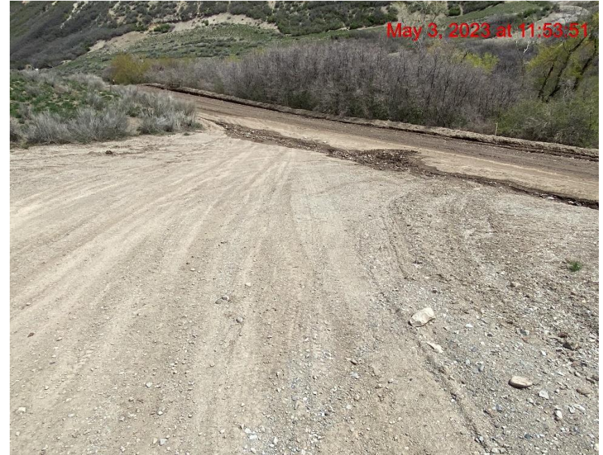
Insufficient Vehicle Tracking BMPs at Location Entrance/Exit – Photo #02863
