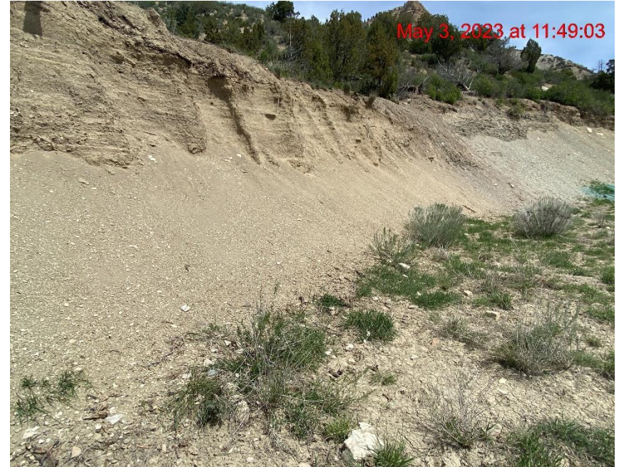
Cut Slope Eroding onto Location – Photo #02855
