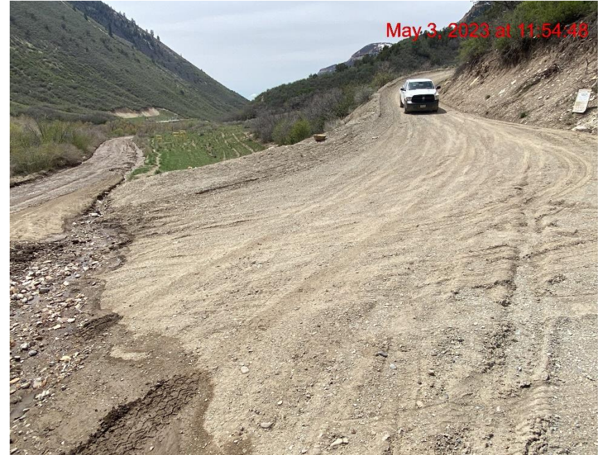
Insufficient Vehicle Tracking BMPs at Location Entrance/Exit – Photo #02866
