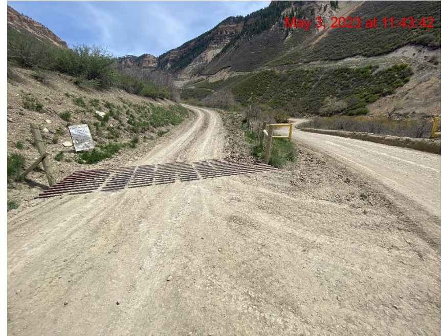
Insufficient Vehicle Tracking BMPs at Location Entrance/Exit – Photo #02849
