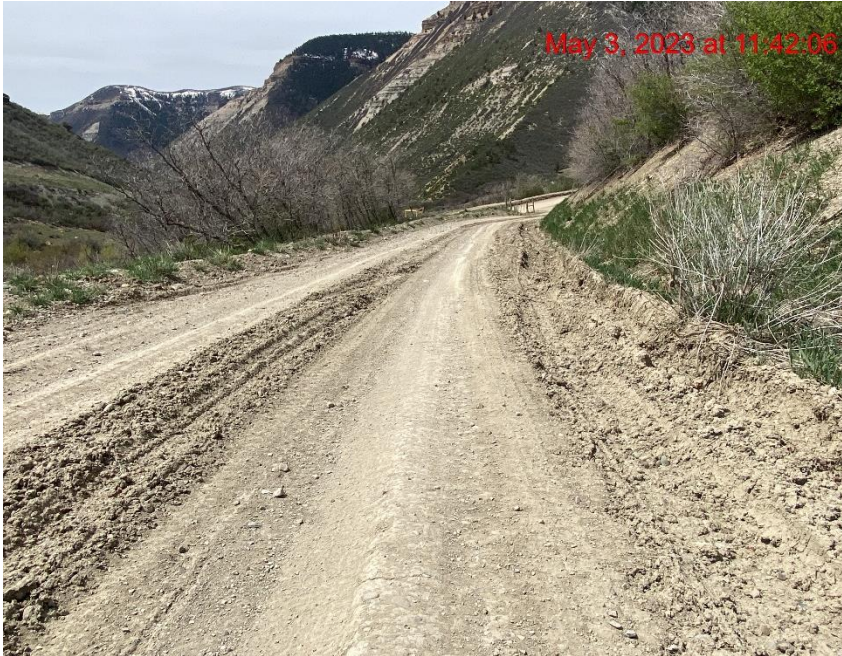
Access Road Lacks Stabilization– Photo #02847
