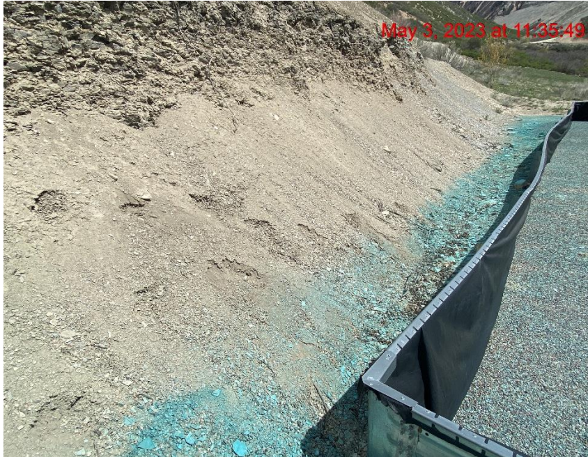
Cut Slope Eroding onto Location – Photo #02838
