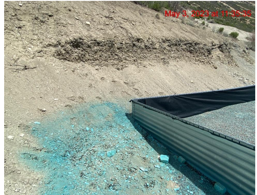
Cut Slope Eroding onto Location – Photo #02838
