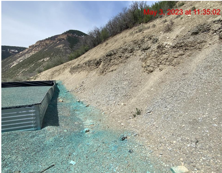
Cut Slope Eroding onto Location – Photo #02836
