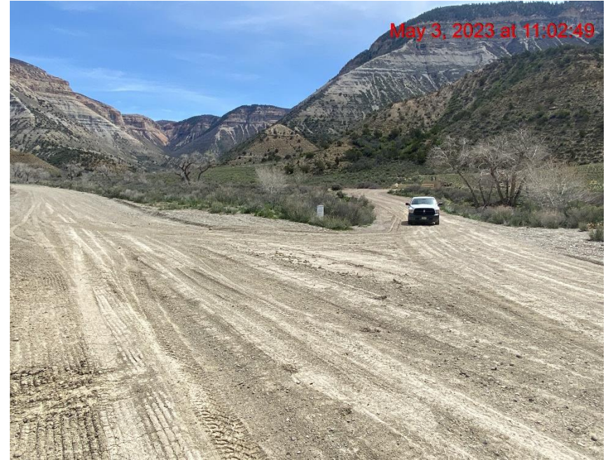
Insufficient Vehicle Tracking BMPs at Location Entrance/Exit – Photo #02830
