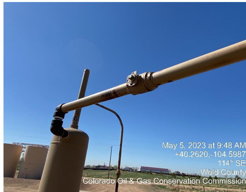
Photo #6 Balon valve on the top side of separator appears to be open going to riser.
