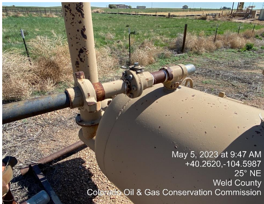
Photo #5 Balon valve appears open going into the separator
