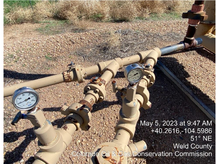
Photo #4 Balon valves appear open at the headed at the separator
