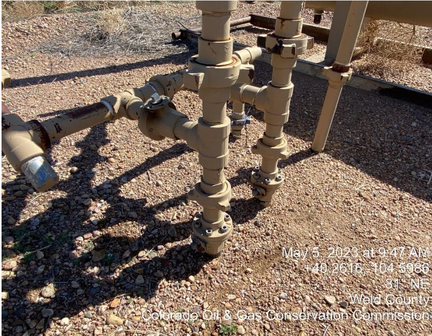
Photo #3 Balon valves appear open at the headed at the separator
