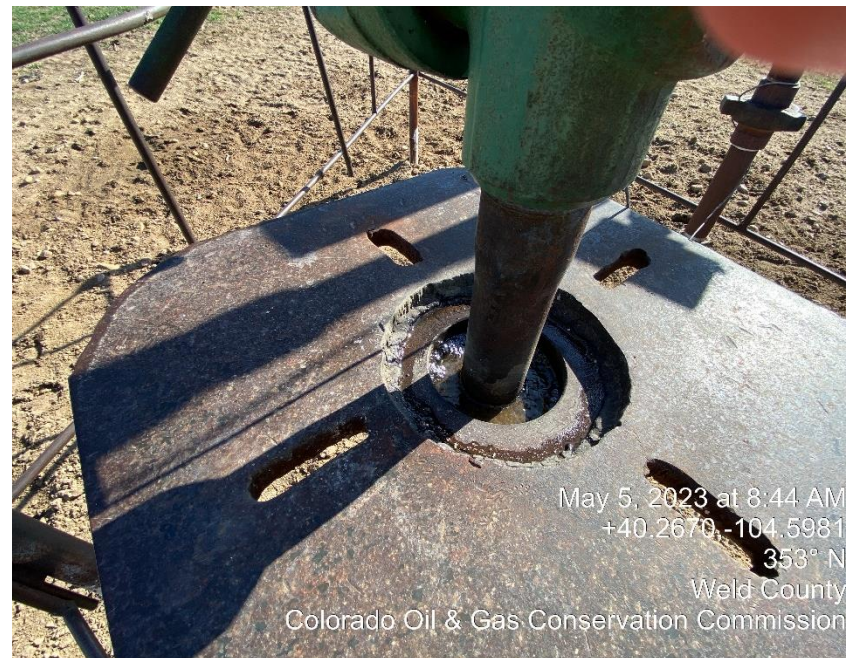
Photo #2 packing leak
