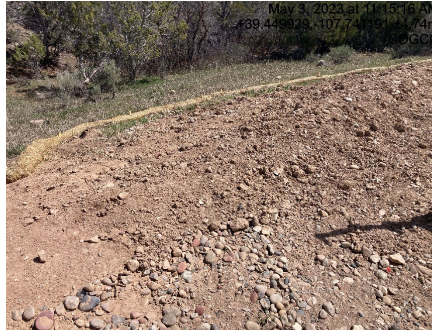
Fill slope lack of stabilization
