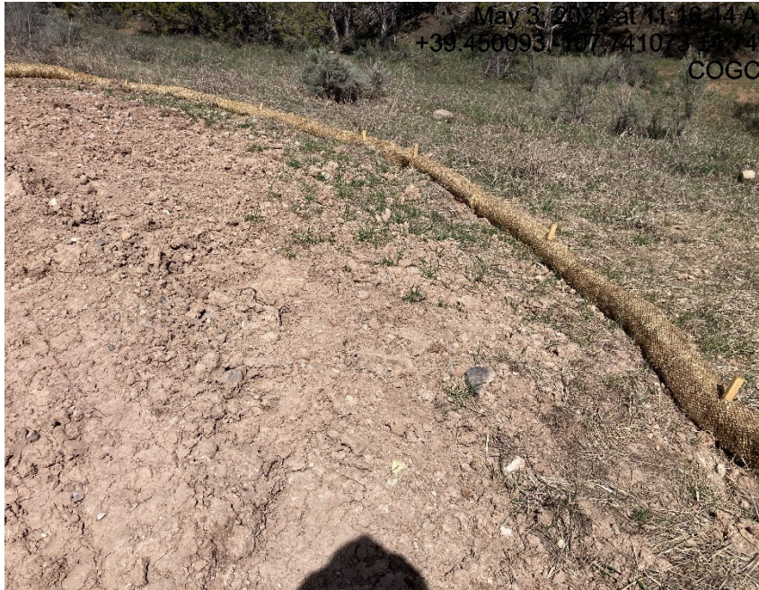
Fill slope lack of stabilization
