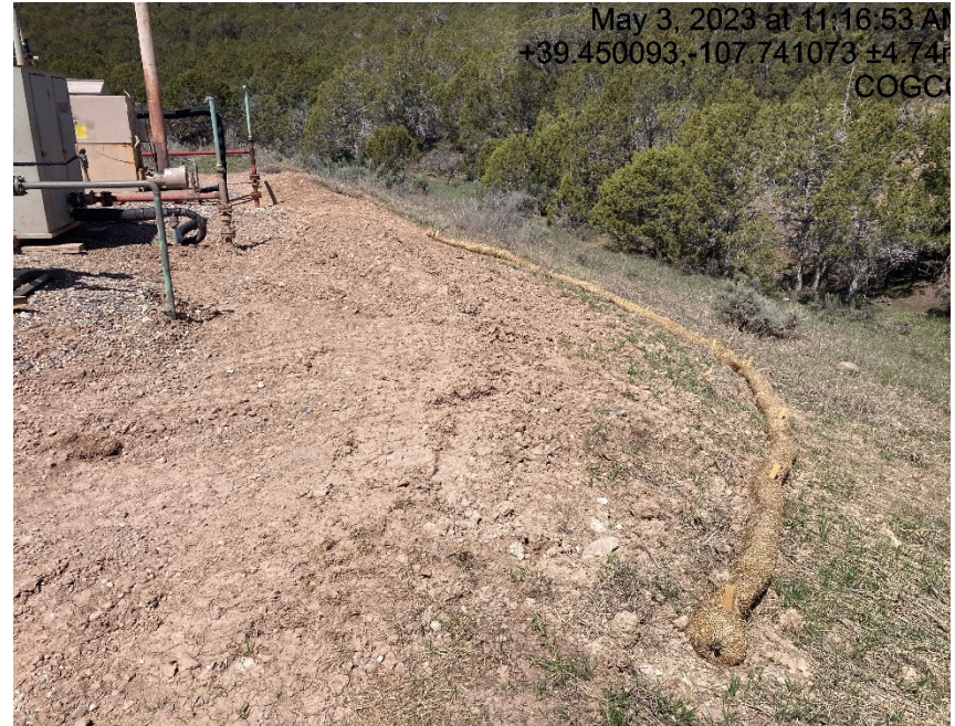
Fill slope lack of stabilization
