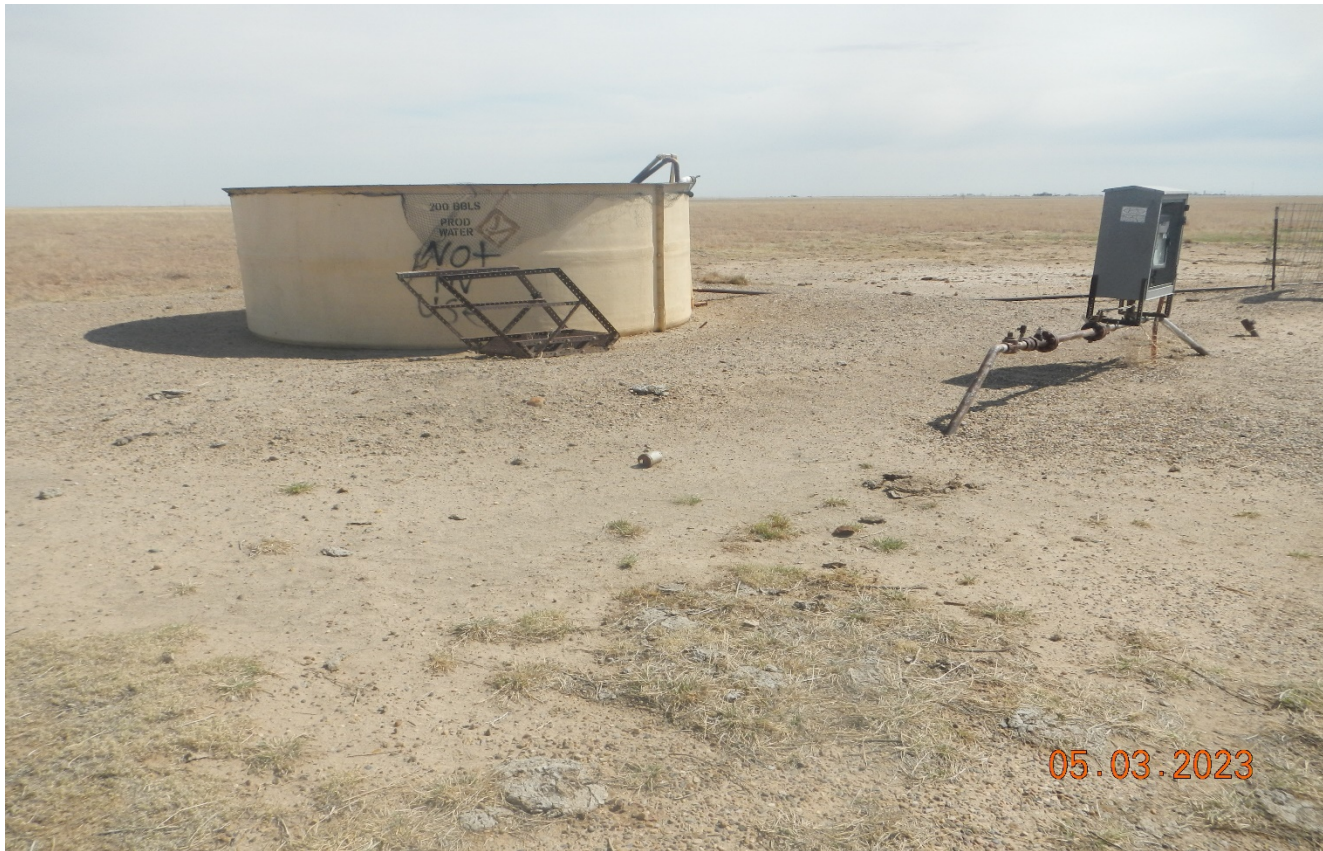
Photo 2. Facing toward the open top tank which still does not have secondary containment.
