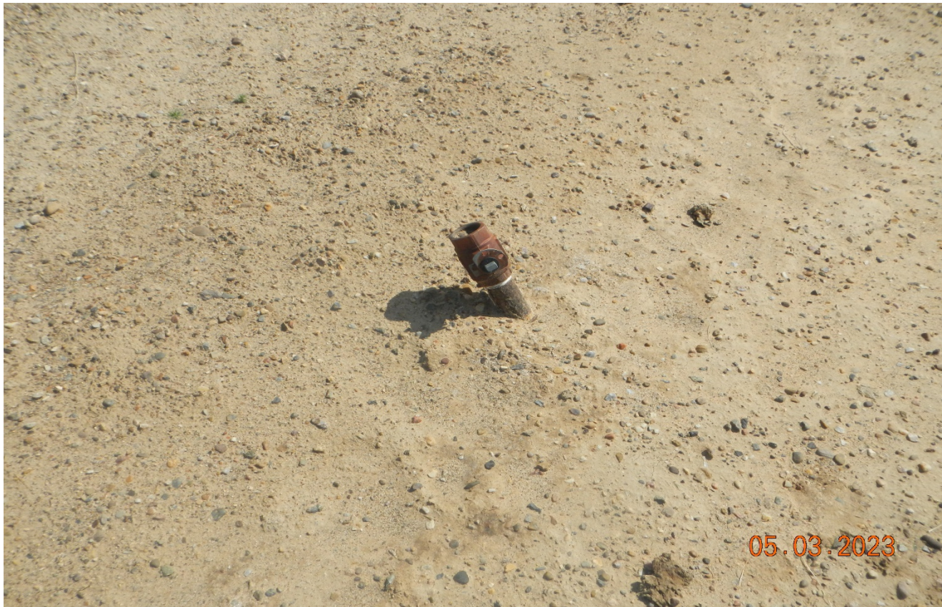
Photo 4. Unused pipe riser still remains with no OOSLAT.
