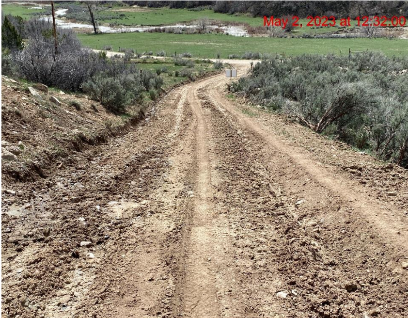
Access Road Lacks Stabilization – Photo #02809
