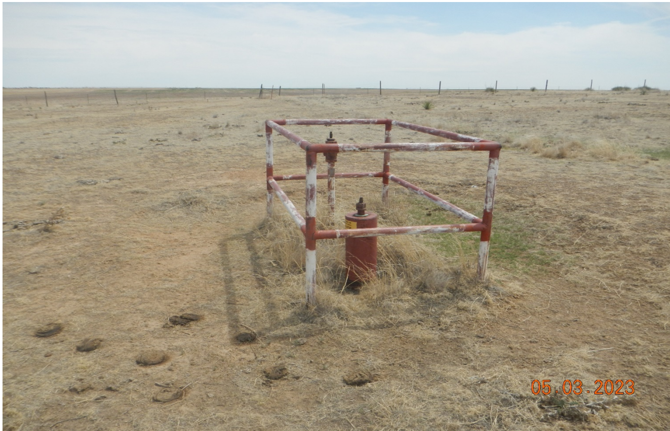
Photo 5. There is another pipeline riser that remains at the south side of the location that has not been removed
