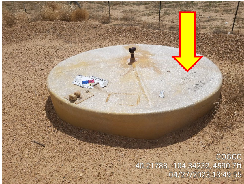
Photo 5 – Water Tank – Labels faded or peeling away
