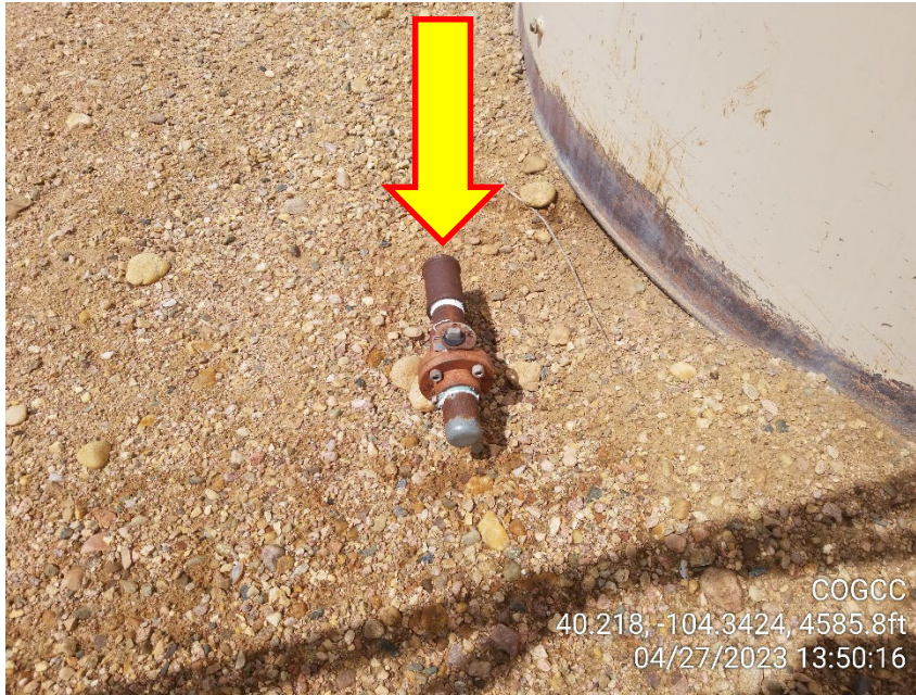
Photo 7 – Unmarked Riser at Crude Oil Tank
