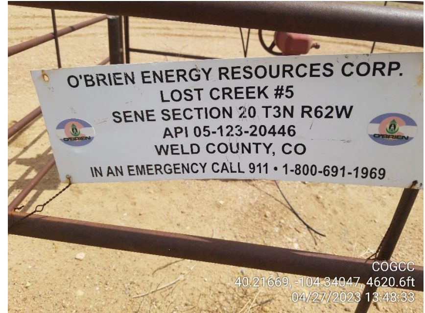
Photo 2 – Wellhead Sign – API is showing wrong Number – Correct API is 05-123-21441
