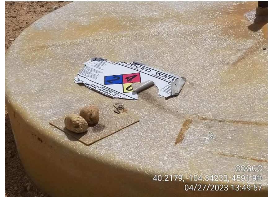
Photo 6 – Label is feeling away – no longer adequate
