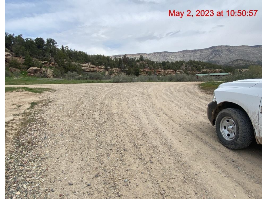
Insufficient Vehicle Tracking BMPs at Location Entrance/Exit – Photo #02746
