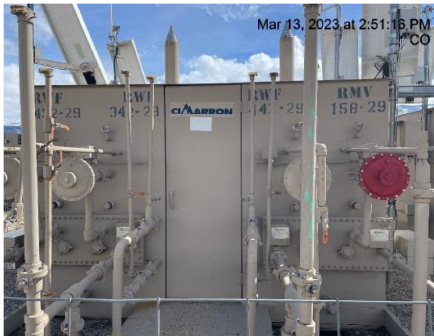
Photo # 2331 From Inspection 708900110 conducted on 03/13/2023 Meter calibration info not conspicuously posted
