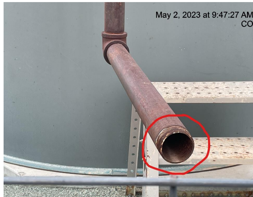
Photo # 6706 Open ended pipe/wildlife hazard
