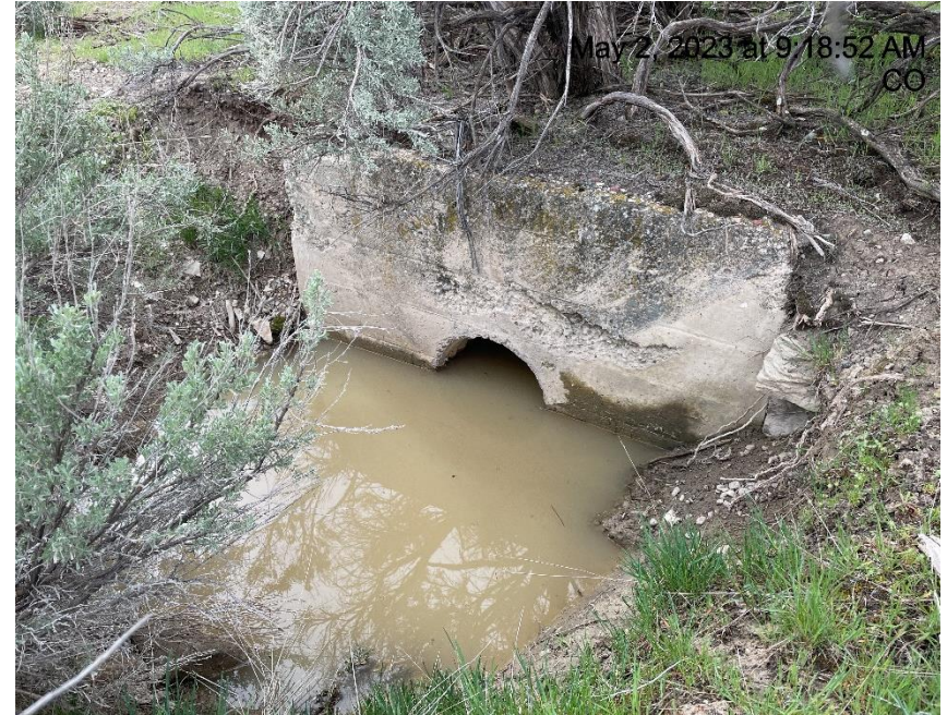
Photo # 6685 Culvert needs maintenance
