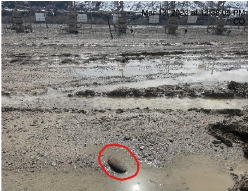
Photo # 2241 From Inspection 708900110 conducted on 03/13/2023 Unmarked deadman
