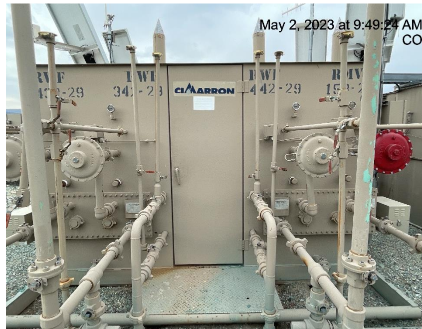
Photo # 6707 Meter calibration info not conspicuously posted
