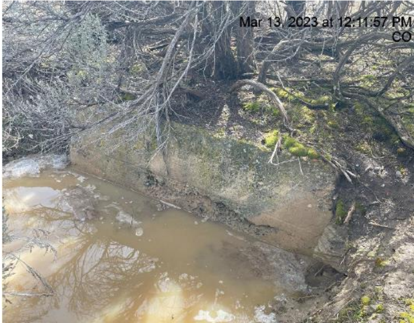
Photo # 2226 From Inspection 708900110 conducted on 03/13/2023 Culvert needs maintenance
