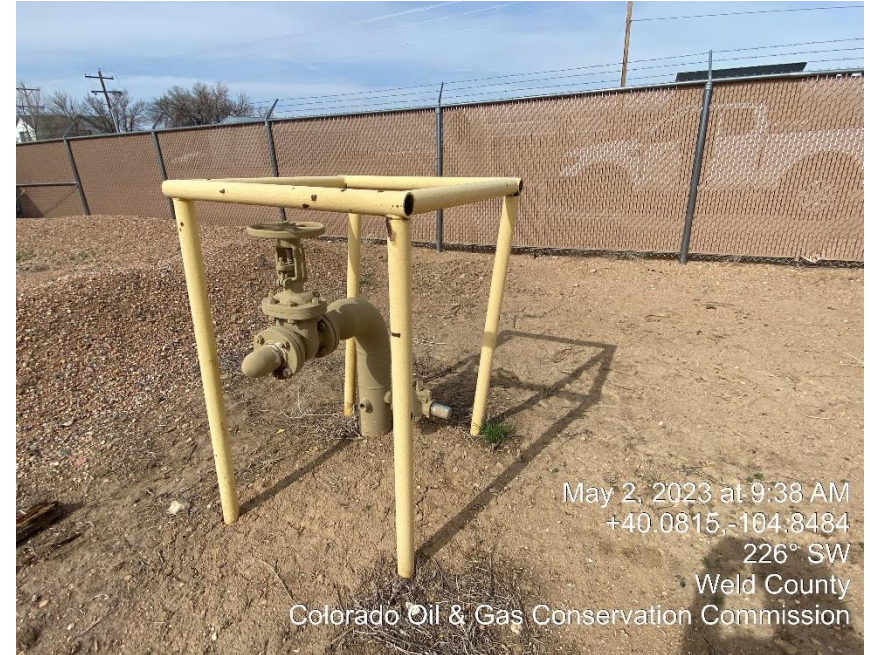
Photo #8 Unmarked Riser
