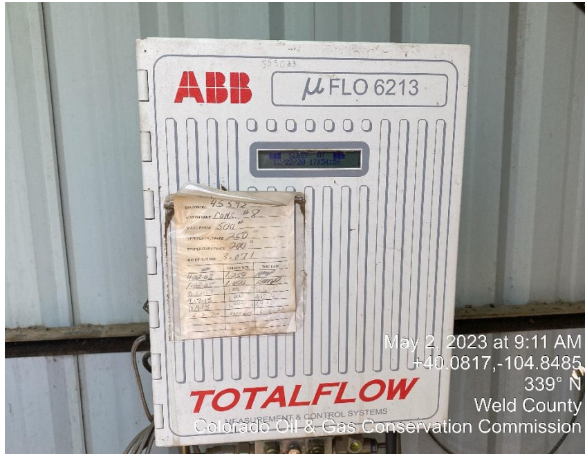
Photo #3 Mechanical Conditions & Meter not calibrated
