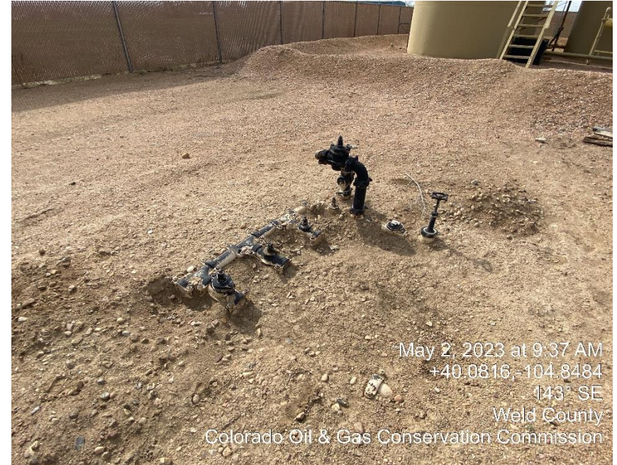
Photo #6 Unmarked Riser
