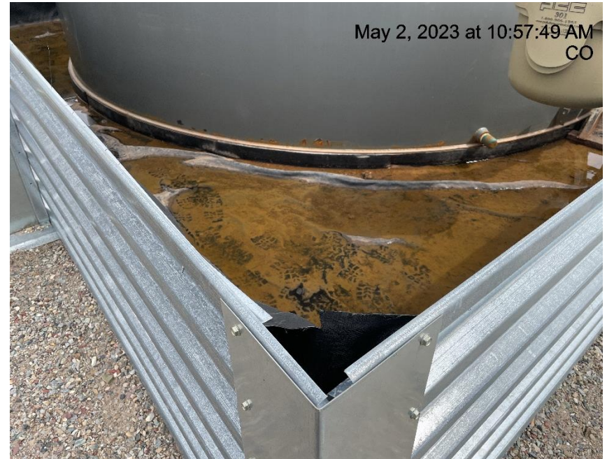
Photo # 6770 Containment needs maintenance
