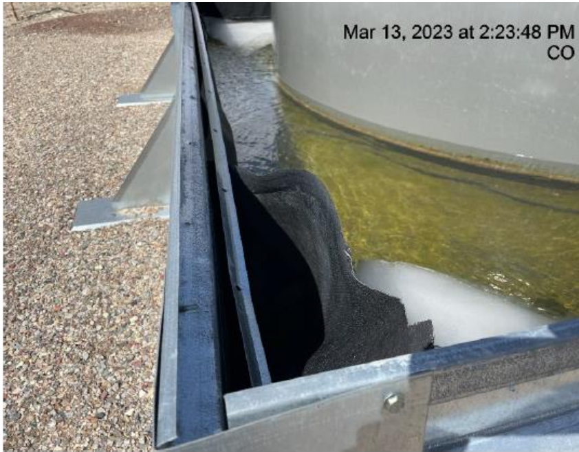
Photo # 2311 From Inspection 708900114 conducted on 03/13/2023 Containment needs maintenance
