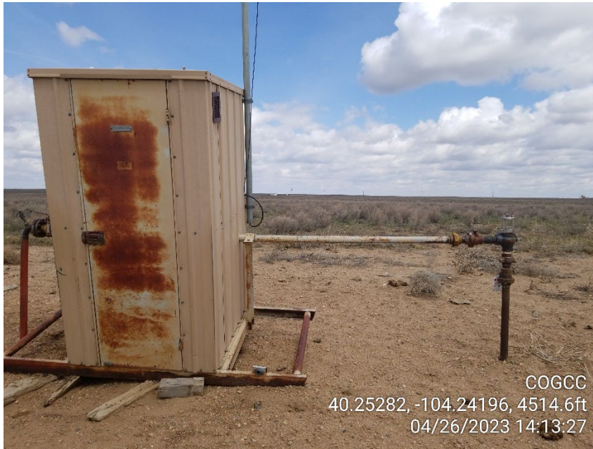
Photo 3 – Gas Meter – LOTO by Sales Operator DCP
