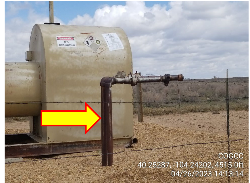
Photo 2 – Unmarked Risers at Separator
