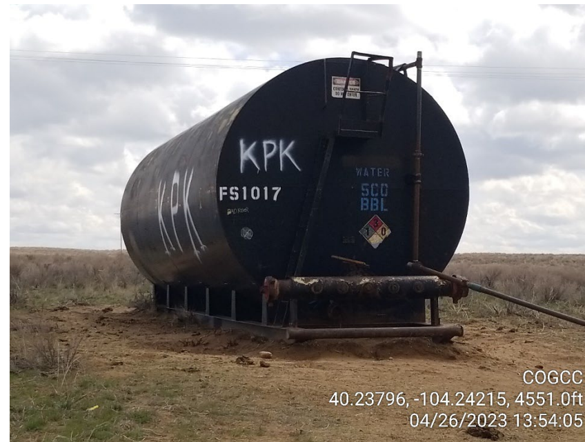
Photo 6 – Temp Water Tank – No Berm
