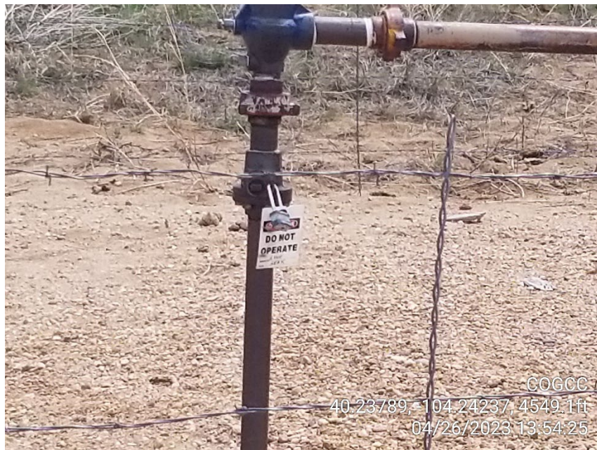
Photo 7 – Sales Line Locked Out/Tagged Out by Sales Operator
