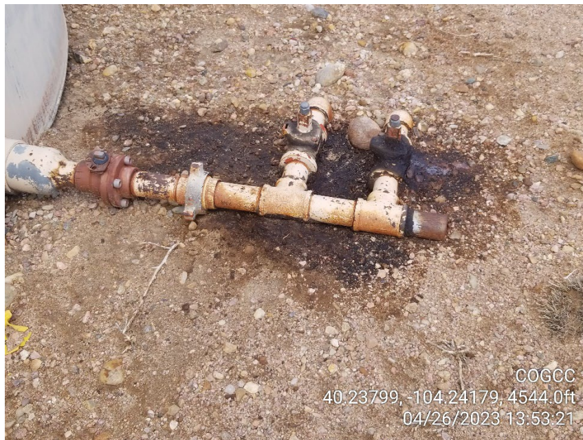
Photo 5 – Stained Soil at Drain Valves at Back side on Tank
