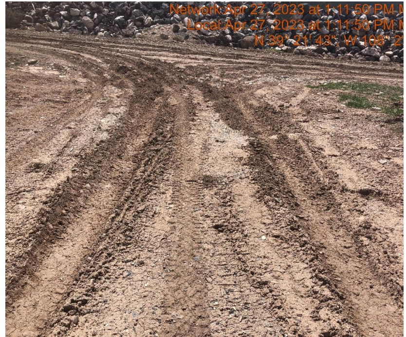
Photo #9775 Insufficient tracking BMP at entrance to location to Minimize the transport of sediment.
