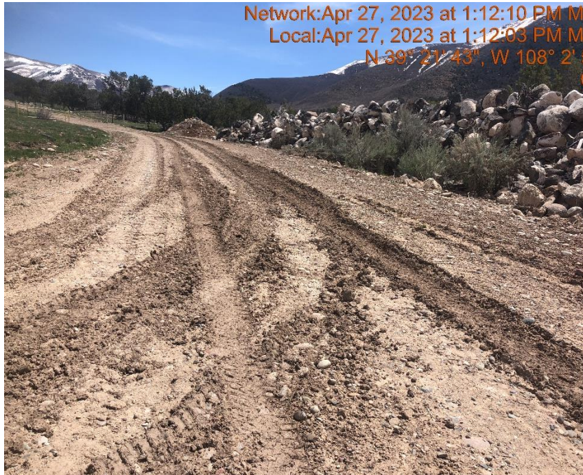
Photo #9776 Insufficient tracking BMP at entrance to location to Minimize the transport of sediment.
