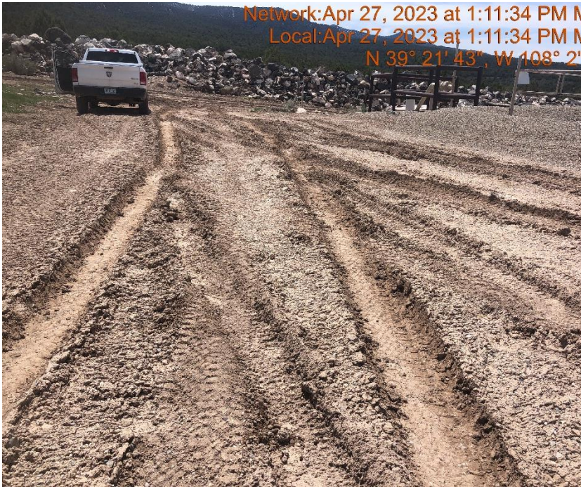
Photo #9774 Location lacks stabilization.
