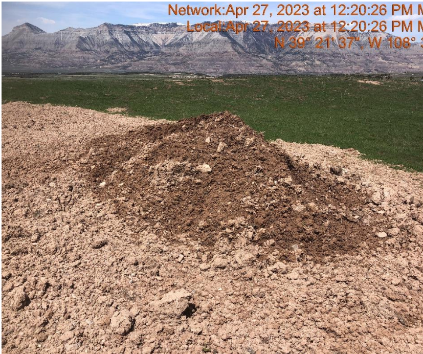
Photo #9743 Insufficient Stock piled soils BMPs.
