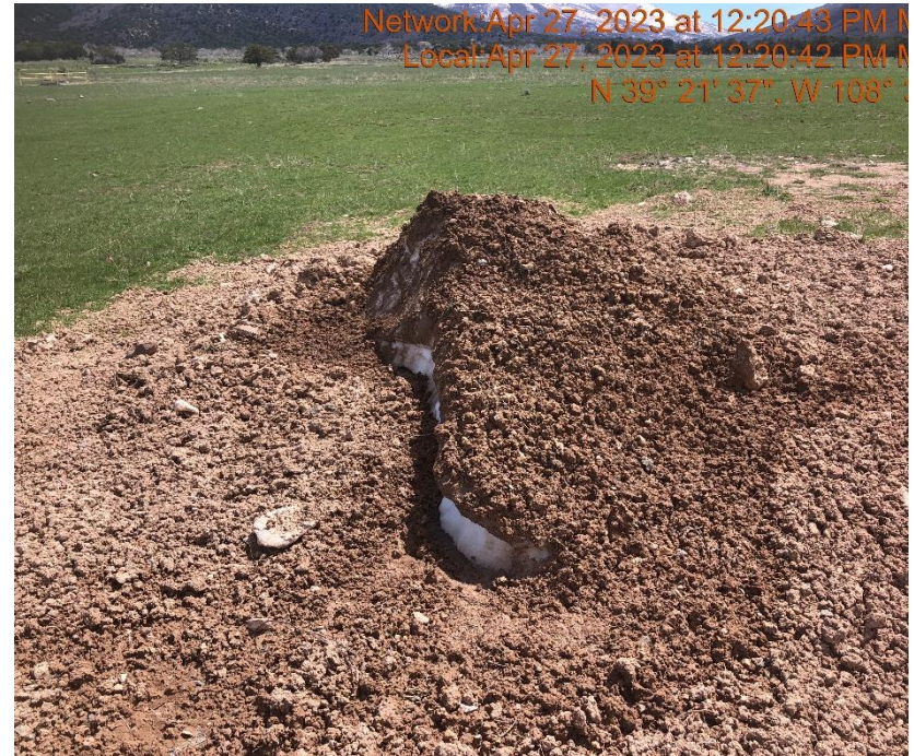
Photo #9744 Insufficient Stock piled soils BMPs.
