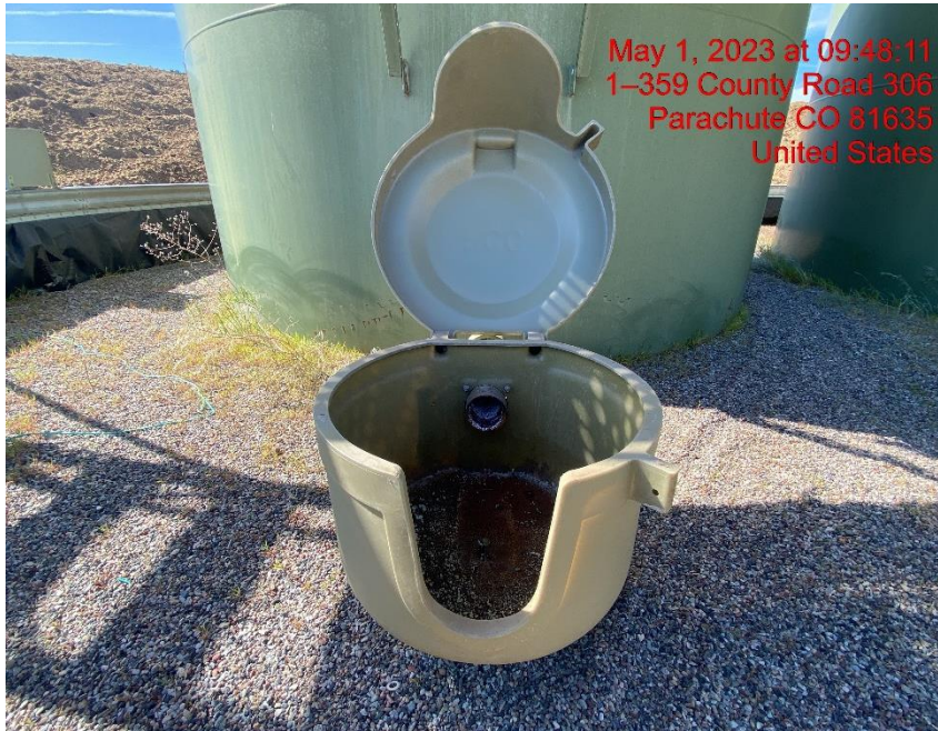
Open-Ended Load Line – Photo #02702
