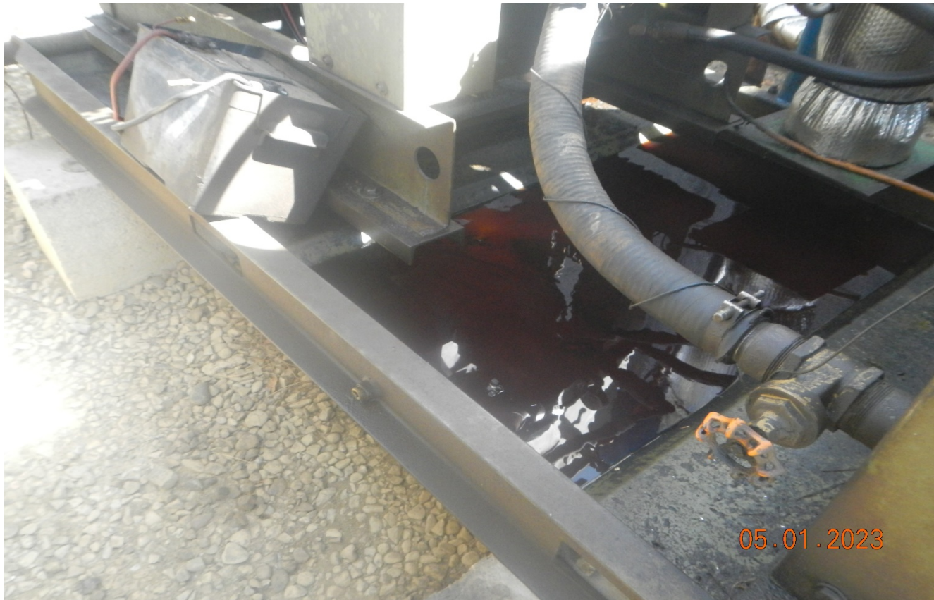
Photo 3. There is oily fluid in the engine skid that needs to be cleaned up.
