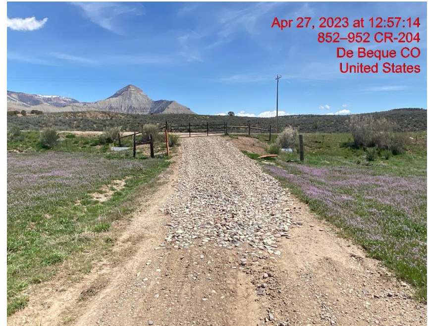
Gravel BMP Installed to Minimize Sediment Transportation – Photo #02659
