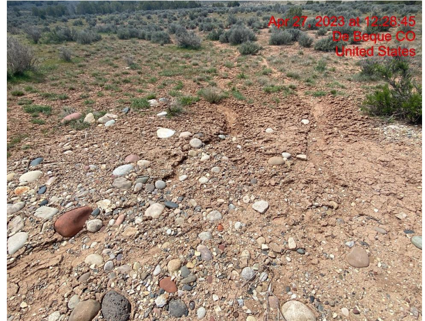
Rill Erosion/Transport of Sediment from Location – Photo #02633
