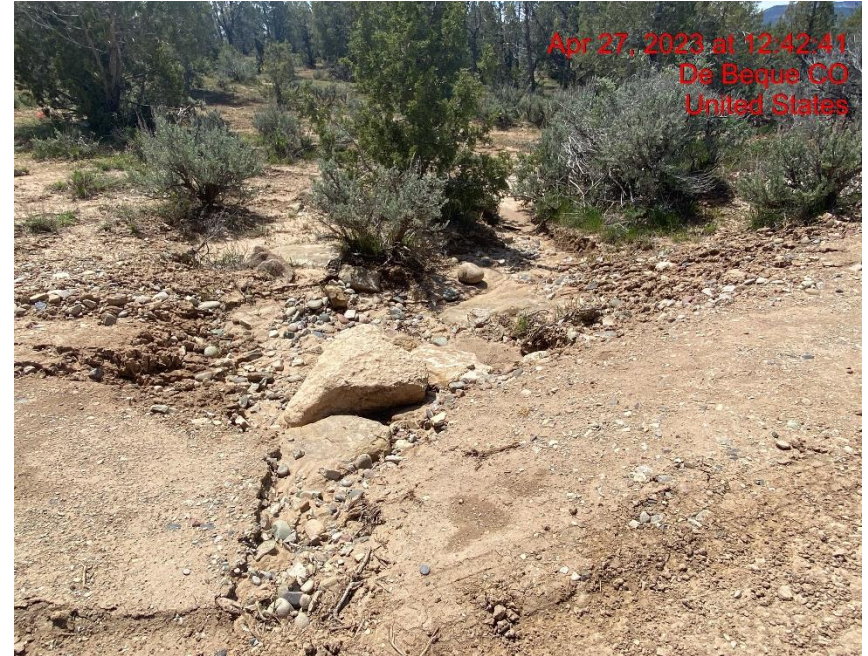
Insufficient BMPs to Minimize Sediment Transportation from Access Road – Photo #02647
