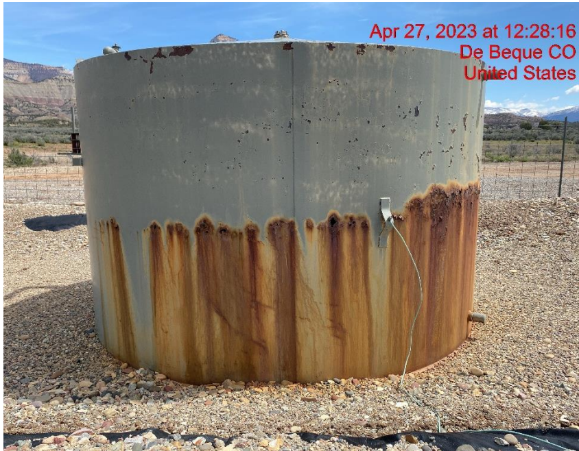
Holes in Produced Water Tank – Photo #02631
