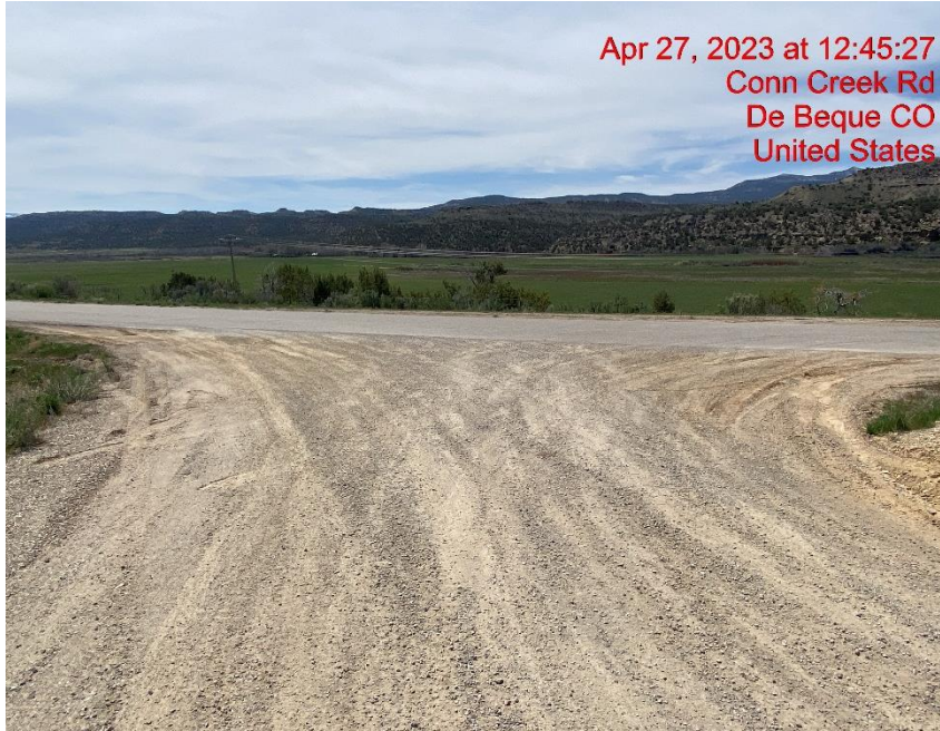
Insufficient Vehicle Tracking BMP – Photo #02648
