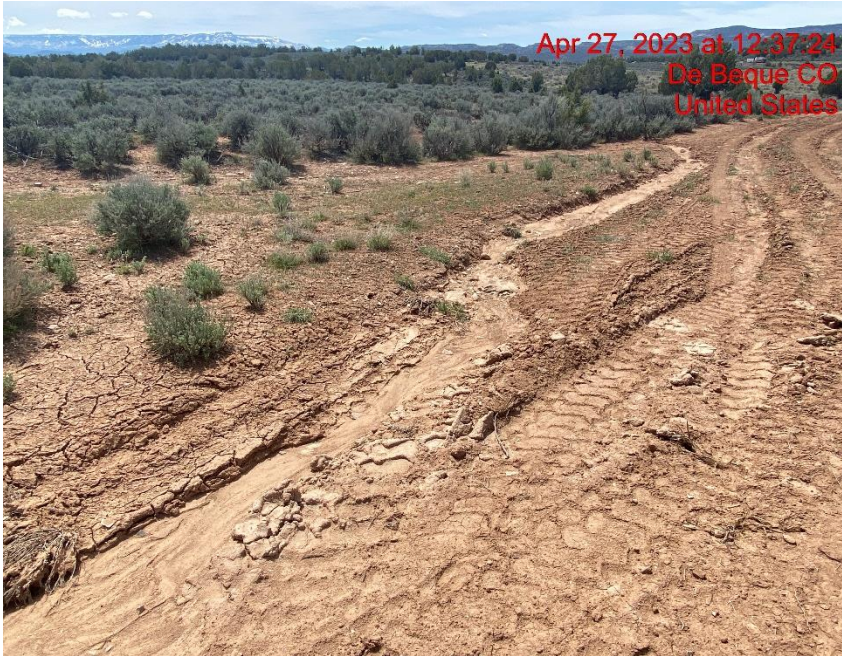
Erosion/Transportation of Sediment from Access Road – Photo #02642
