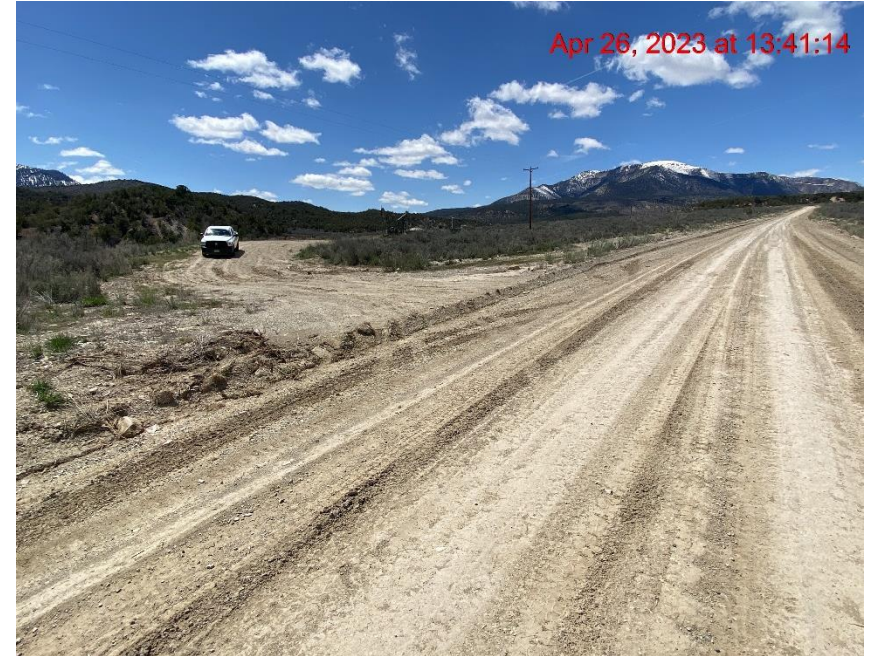
Insufficient Vehicle Tracking BMP at Location Entrance/Exit – Photo #02626
