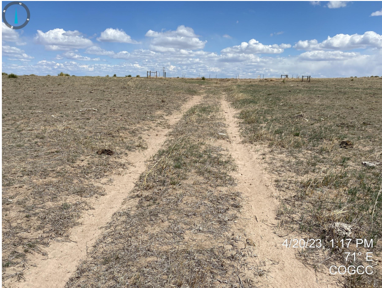
Photo 1. It does not appear the access/lease road has been reclaimed or contoured to reflect pre-disturbance conditions with rutting evident.
