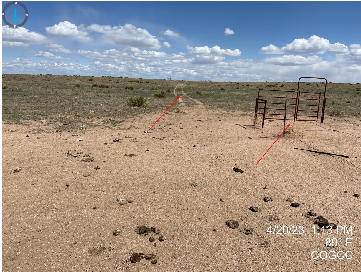
Photo 7. Facing east from the lease road entrance. Photo illustrates that the access road does not appear to have been reclaimed and is not progressing towards final reclamation standards. Also pictured, equipment (e.g. fencing) remains around the former tank battery location.
