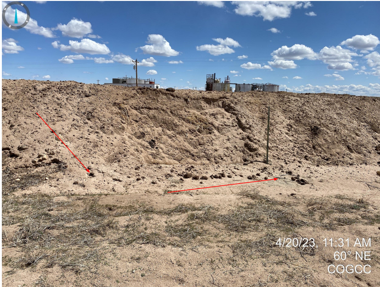
Photo 7. South pit walls do not appear to be properly stabilized with evidence of unconsolidated material and sediment deposition at the base of the wall.
