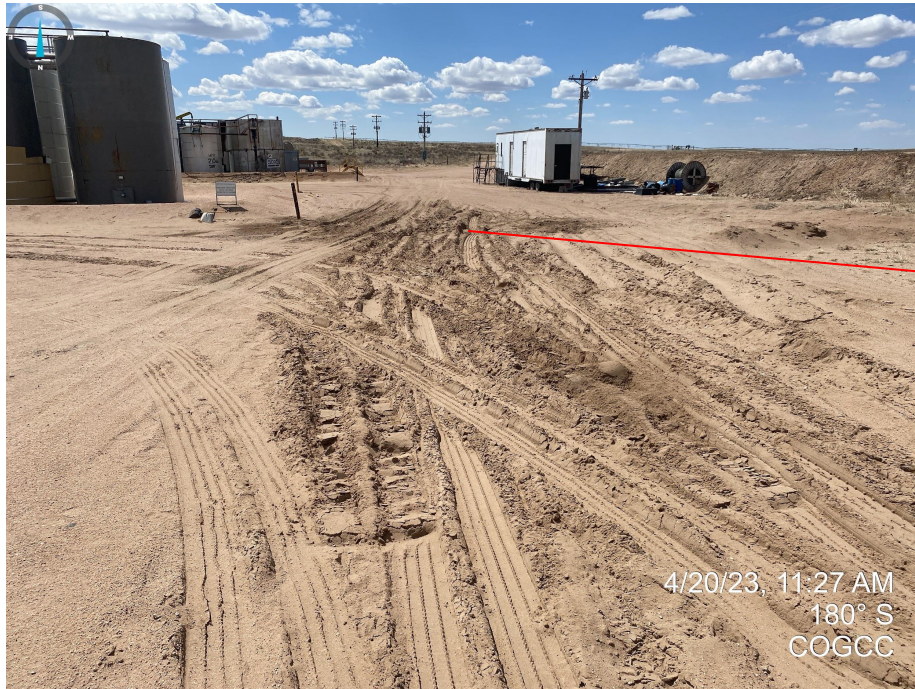
Photo 1. Production areas don't appear to be properly stabilized with evidence of deep rutting.
