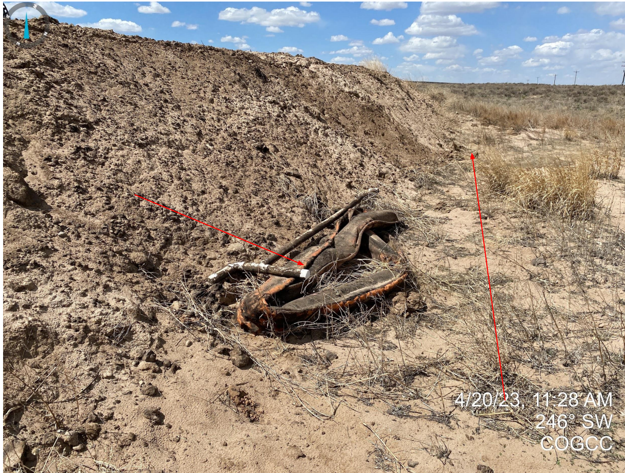
Photo 2. Hydrocarbon soaked filter media observed on the north side of the pit will need to be properly disposed of, including any stained soil. Also pictured, pit walls do not appear to be properly stabilized with evidence of unconsolidated material and sediment deposition at the foot of the wall.
