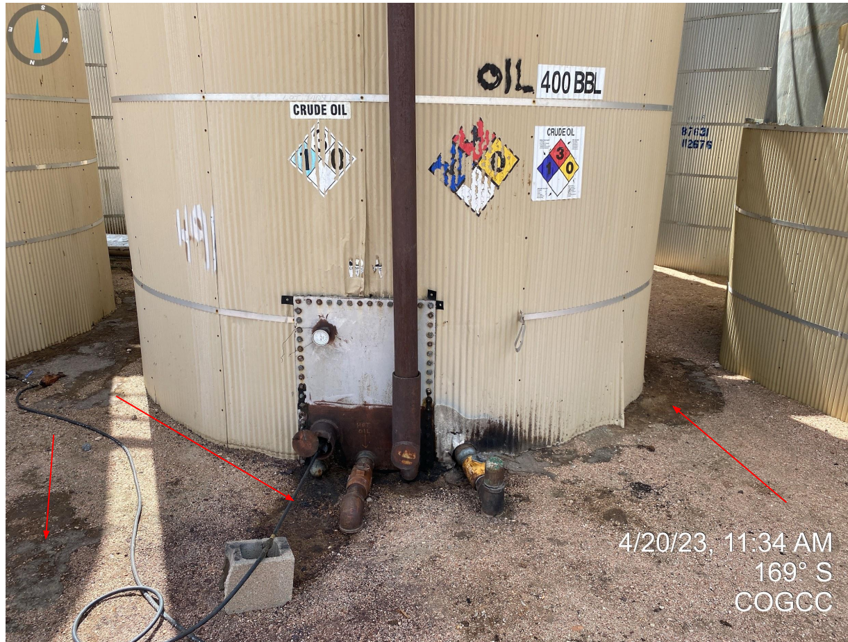
Photo 10. Stained soil observed around equipment. The operator is required to clean up all stained soil (including areas not identified in inspection photos) per Rule 912.b. Additionally, Operator shall perform maintenance on equipment, fittings, connections, etc to ensure good mechanical condition per Rule 608.e.
