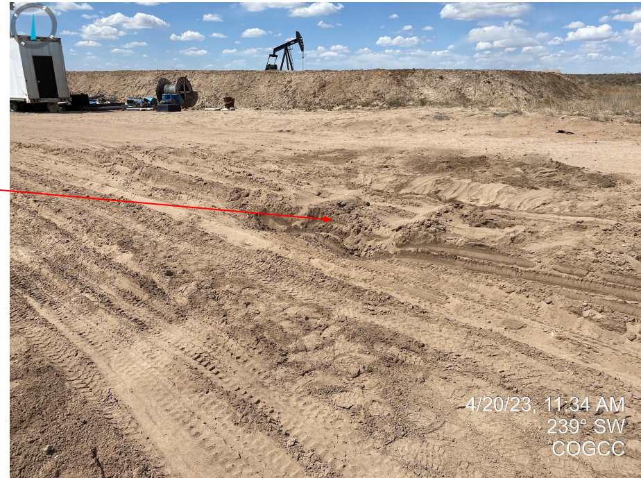
Photo 1. Production areas don't appear to be properly stabilized with evidence of deep rutting.
