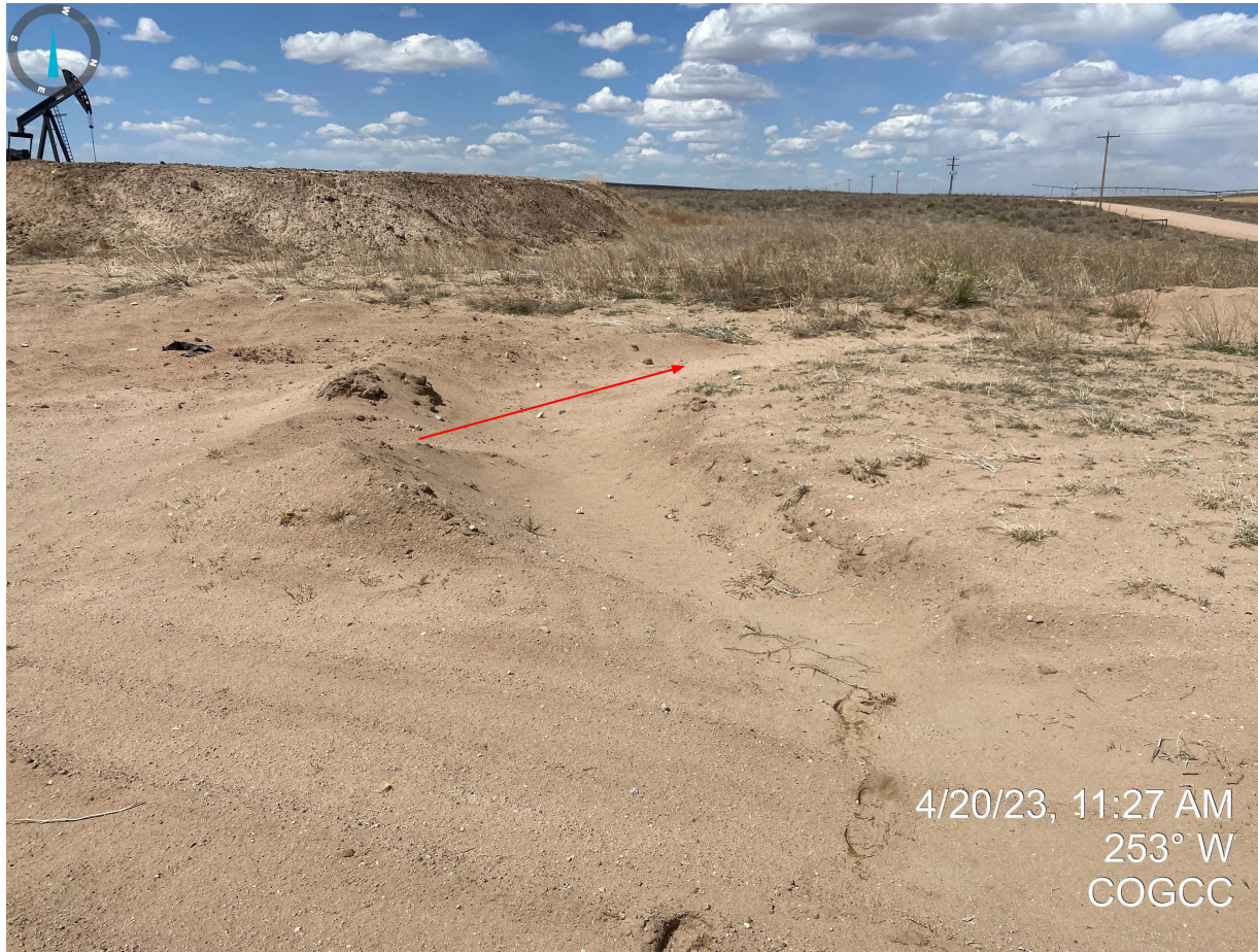
Photo 21. Stormwater ditch/diversion was constructed near the northwest portion of the location's entrance leading to off-site sediment transport into adjacent bar ditch. It does not appear that a properly engineered sediment basin was constructed in this area as it is a natural low point on the location. More robust stormwater BMPs must be implemented to manage stormwater run on and run off to prevent further degradation to adjacent land.
