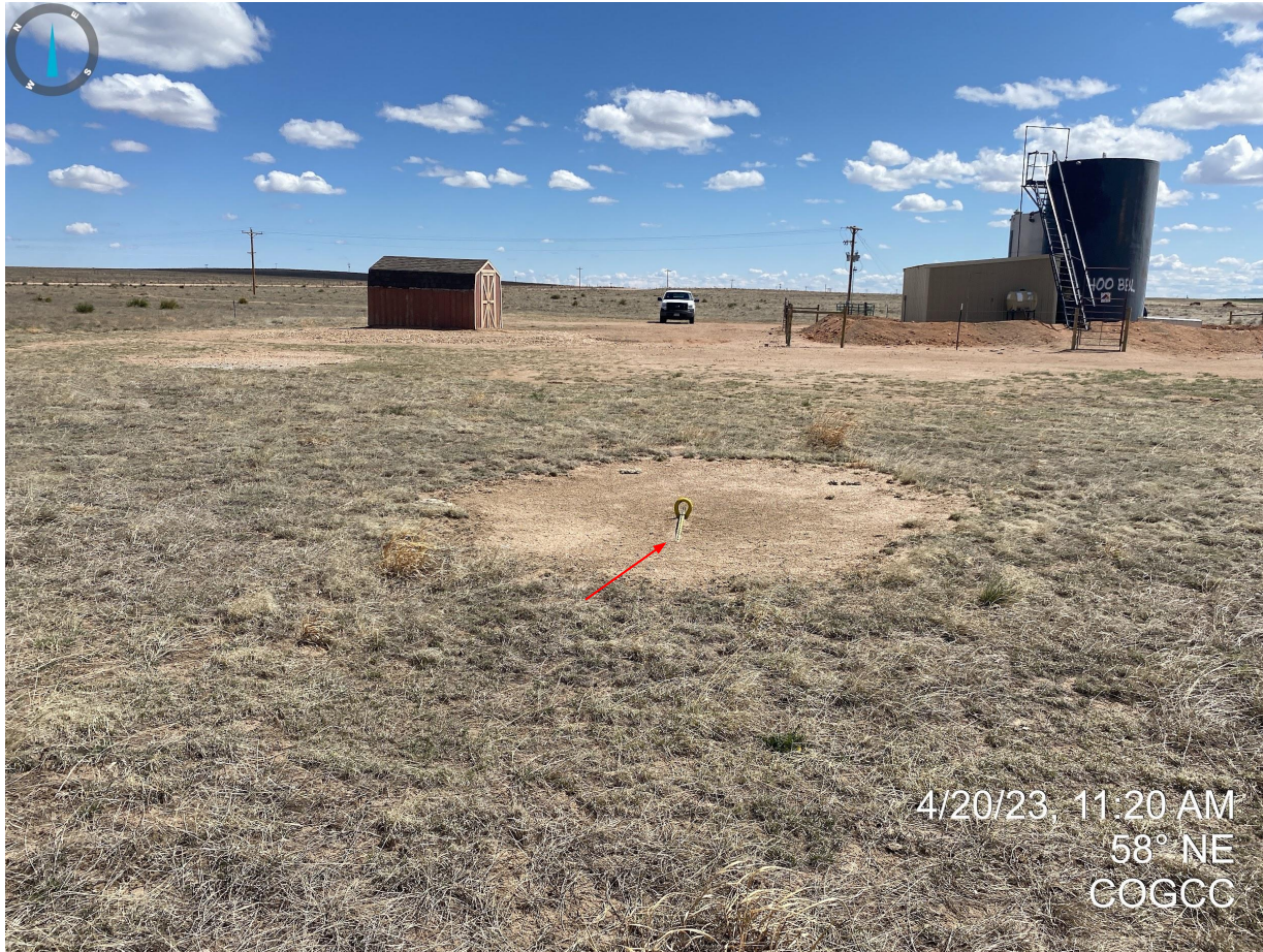
Photo 4. Guy line anchors not properly marked per Rule 603.j
