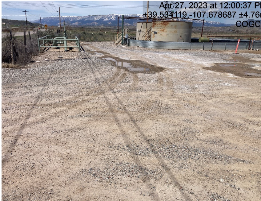
Lack of stabilization/compaction
