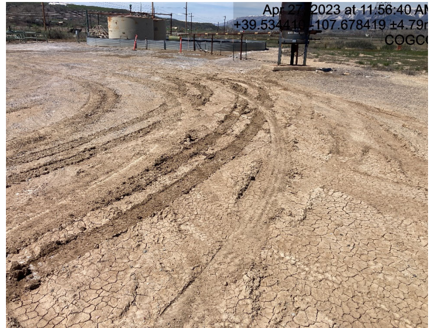
Lack of stabilization/compaction
