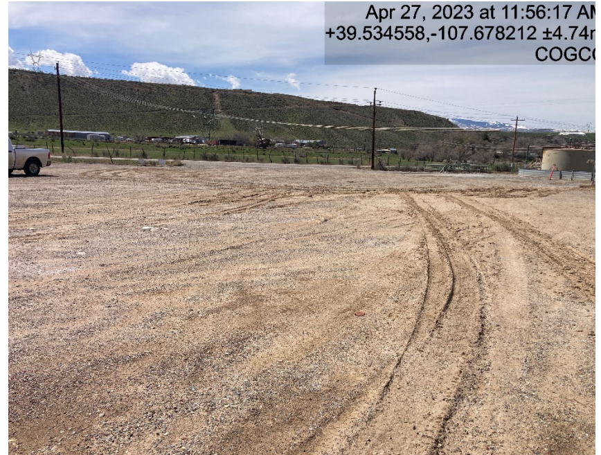
Lack of stabilization/compaction
