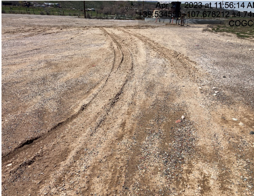
Lack of stabilization/compaction
