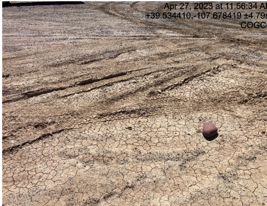
Lack of stabilization/compaction
