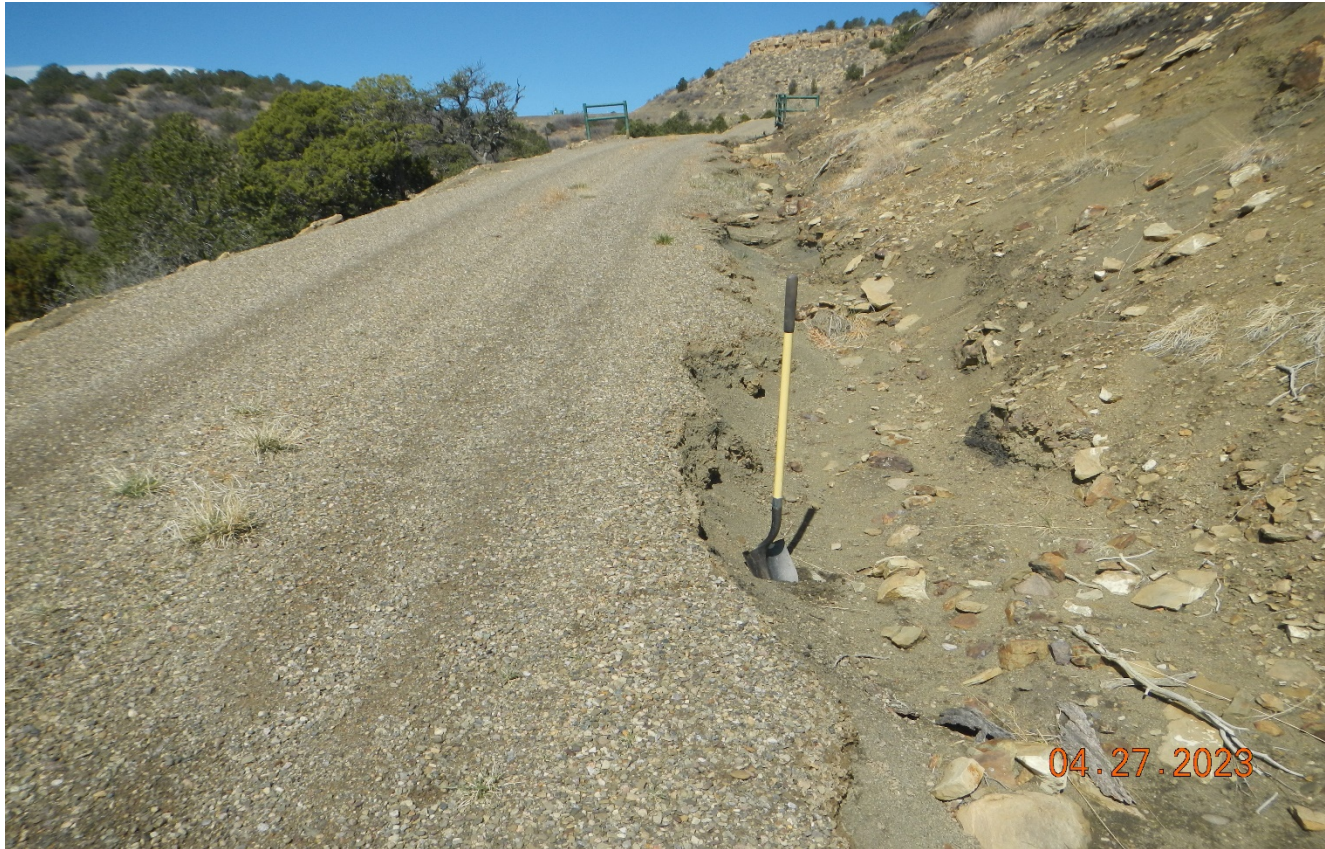
Photo 4. Facing northwest along the access road. Shovel placed in erosion channel for scale.
