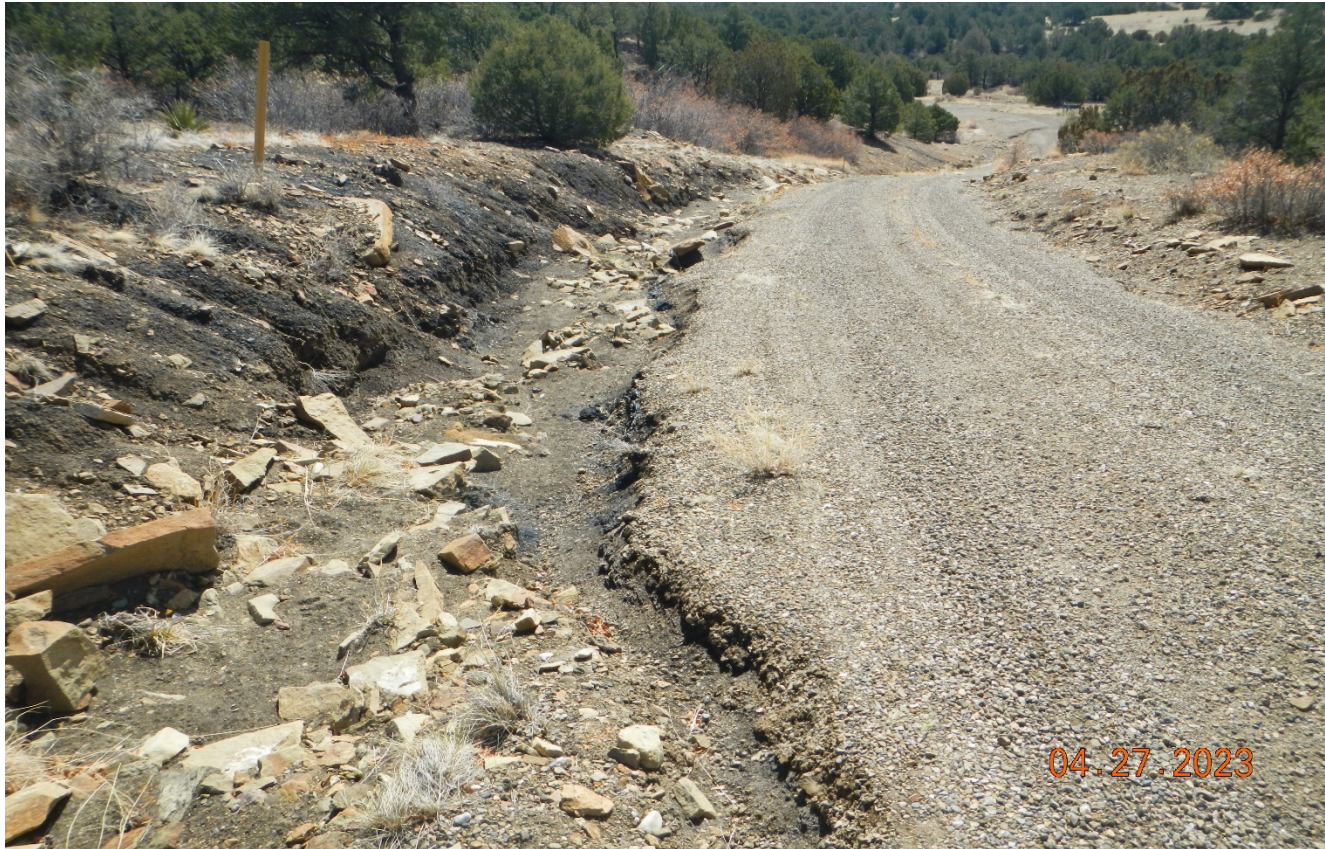
Photo 3. Facing back southeast along the access road. There is erosion along the roadside and stormwater is not diverted and runs down the entire length of the access road.
