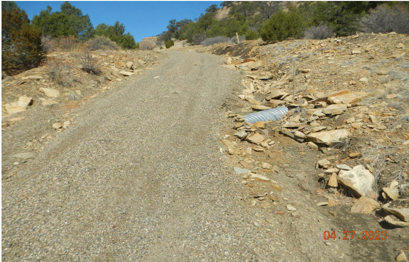
Photo 2. This culvert is filled in with sediment and there were no other culverts observed . Stormwater is all the way down the roadside causing erosion.
