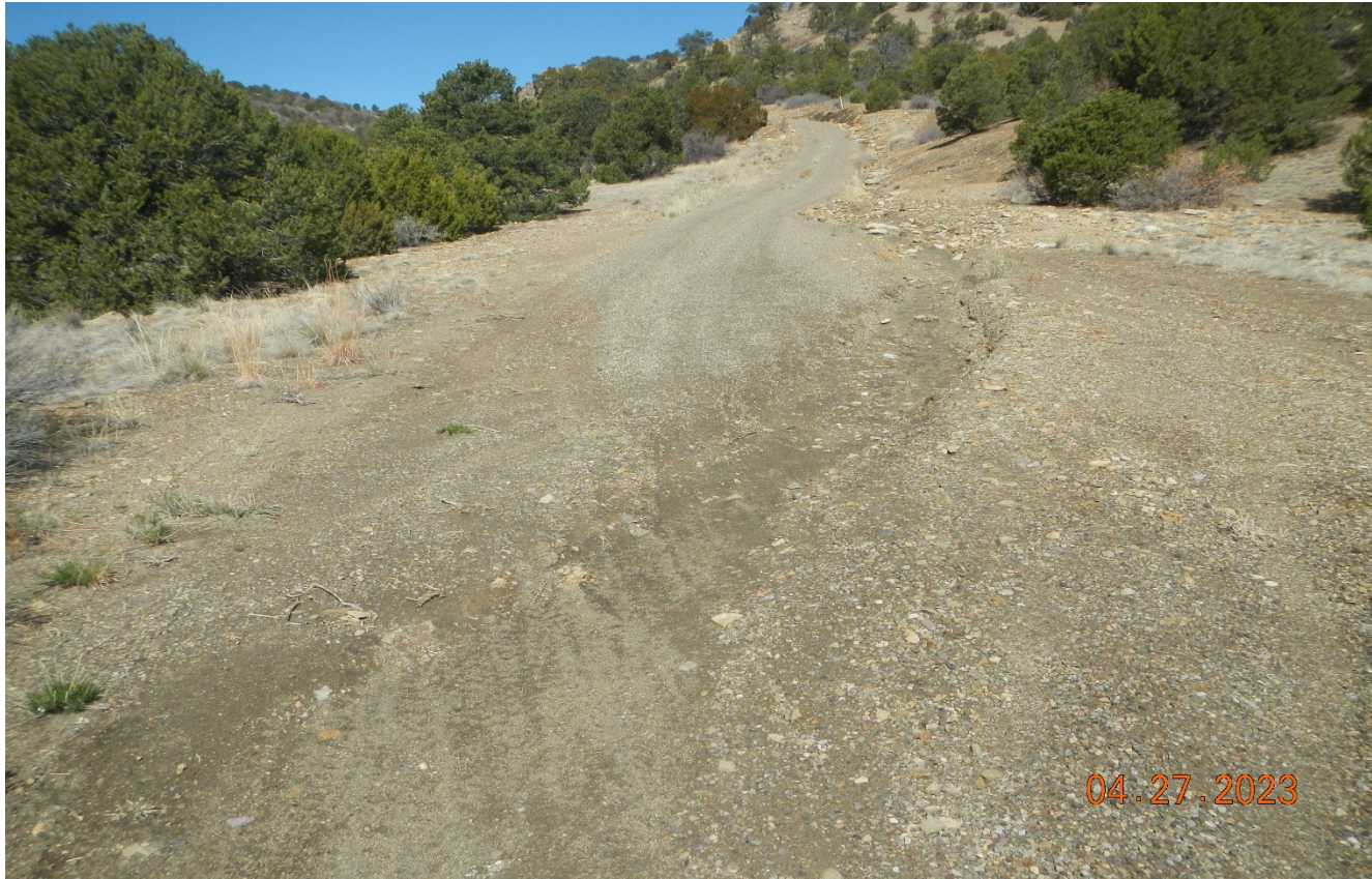
Photo 1. Facing northeast at the access road. Stormwater is directed all the way down the roadside causing erosion of the road.
