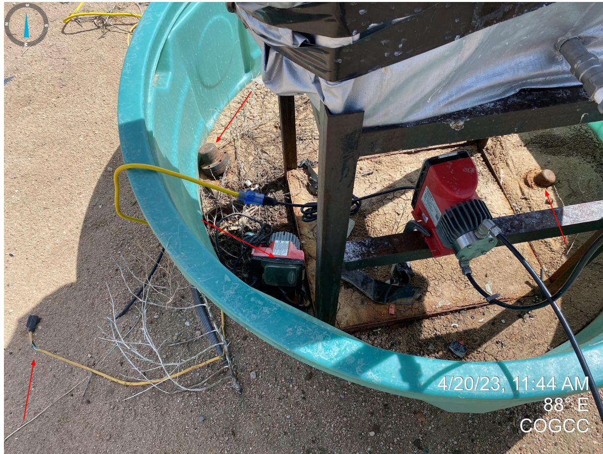
Photo 4. Close-up of day tank near wellhead. Photo illustrates unused equipment and no wildlife netting installed around secondary containment.
