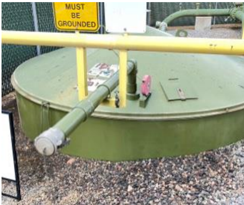
Photo #3. Produced water tank with impacted gravel.
