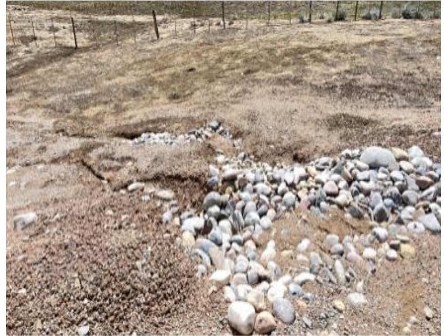
Photo #2. View of erosion on run-downs.
