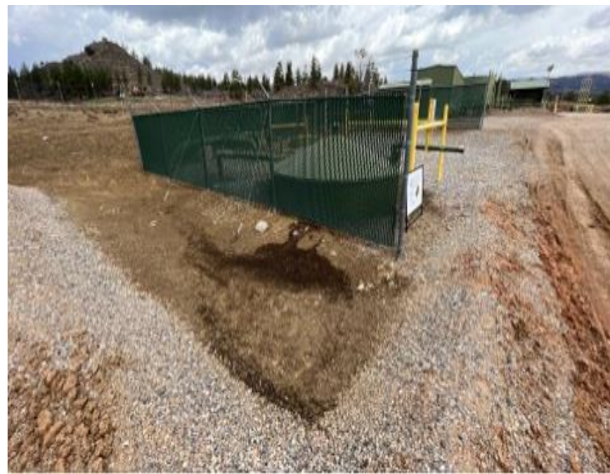
Photo #4. Impacted area from produced water tank spill.
