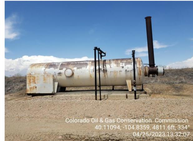
**Photo 12 Horizontal Heater Treater.**
