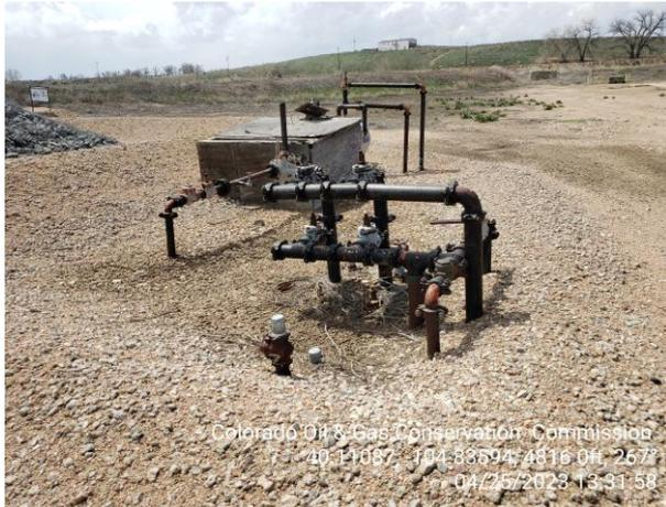
**Photo 11 Flow line manifold.**
