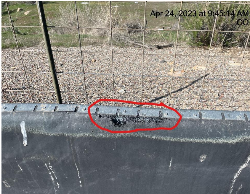
Photo # 6130 Containment liner needs maintenance
