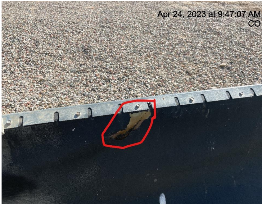
Photo # 6135 Containment liner needs maintenance
