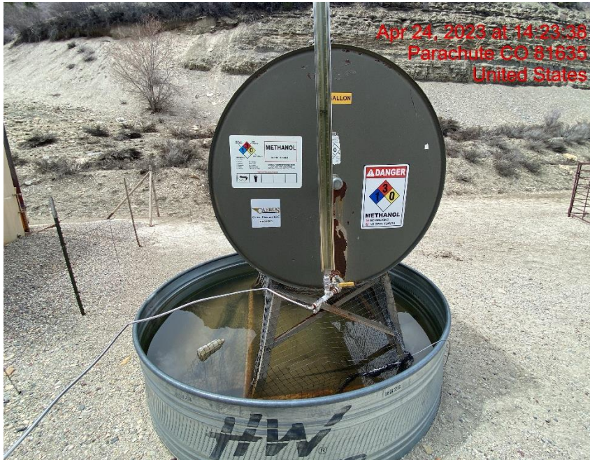
Inadequate Containment Capacity – Photo #02529
