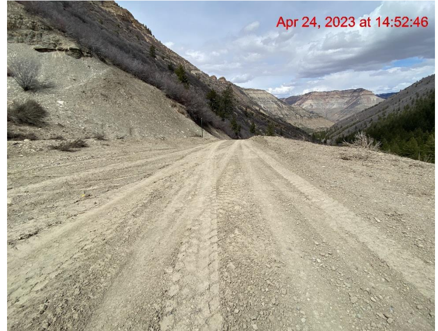
Inadequate Vehicle Tracking BMPs at Location Entrance – Photo #02536
