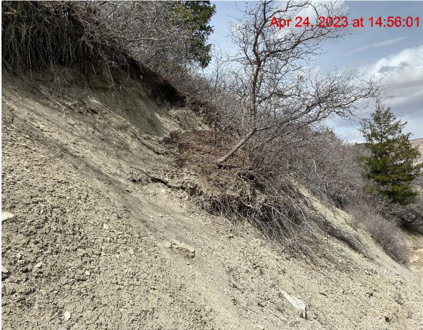
Slope Erosion onto Access Road – Photo #02544
