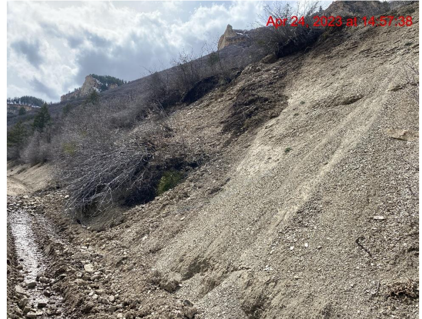
Slope Erosion onto Access Road – Photo #02546
