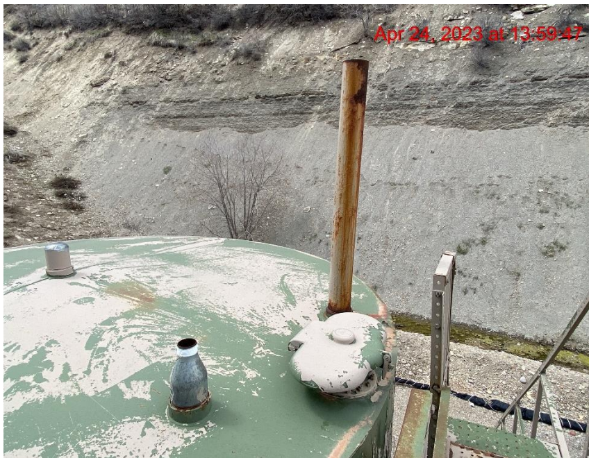
No Wildlife Protection Equipment Installed – Photo #02518
