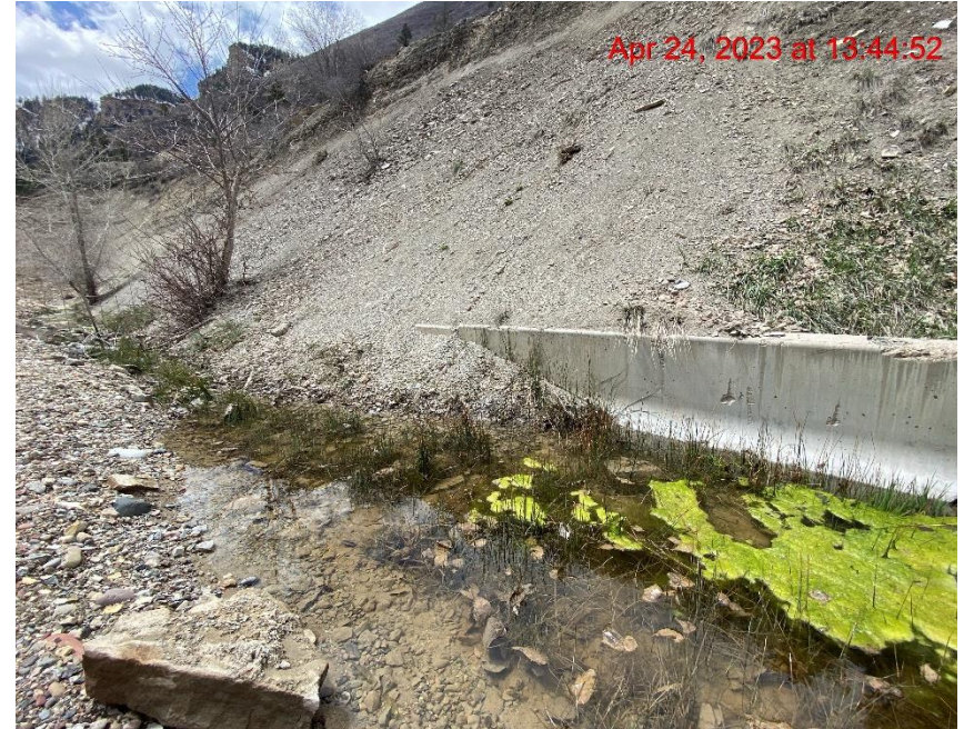
Slope Erosion has Overrun Retaining Wall – Photo #02514
