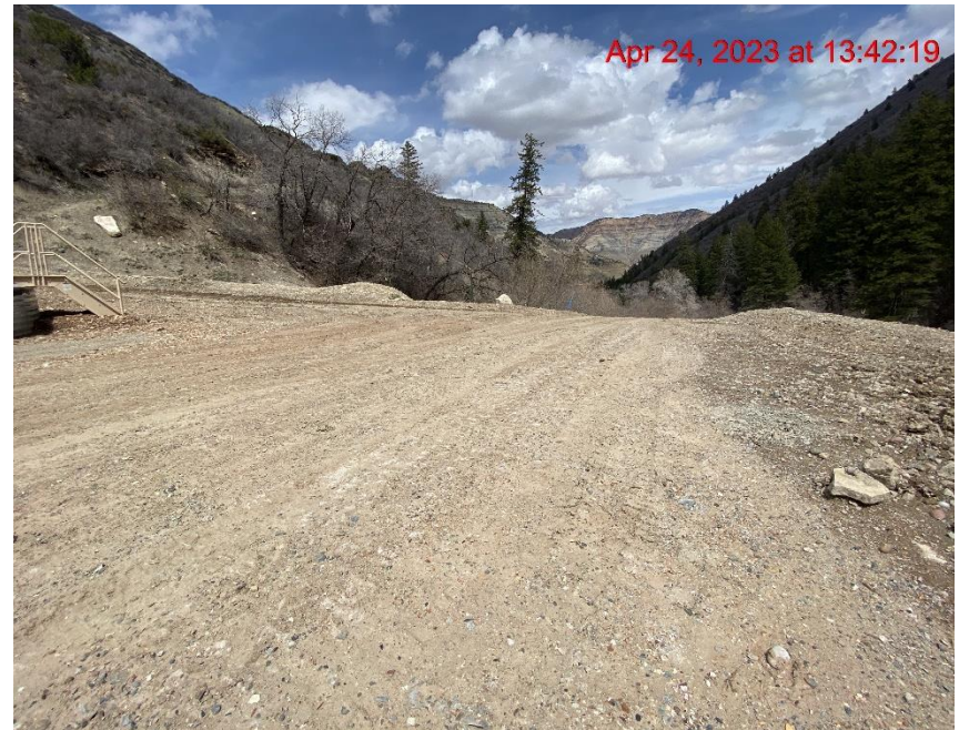
Inadequate Vehicle Tracking BMPs at Location Entrance – Photo #02512
