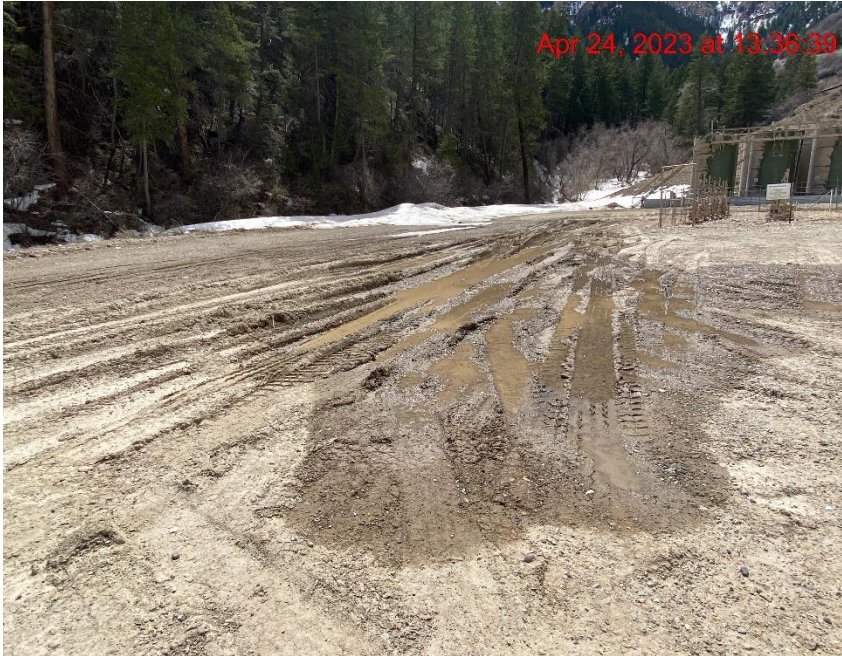
Lack of Stabilization – Photo #02500
