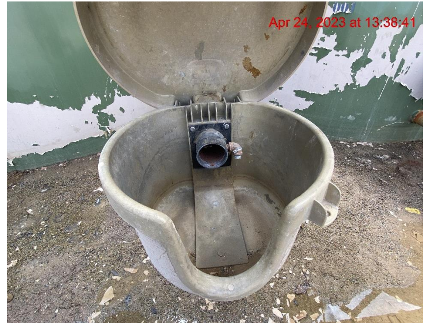
Open-Ended Load Line – Photo #02505
