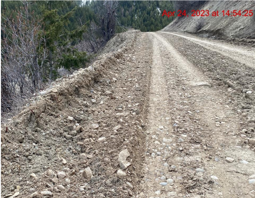
Access Road Degradation/Transportation of Sediment – Photo #02540
