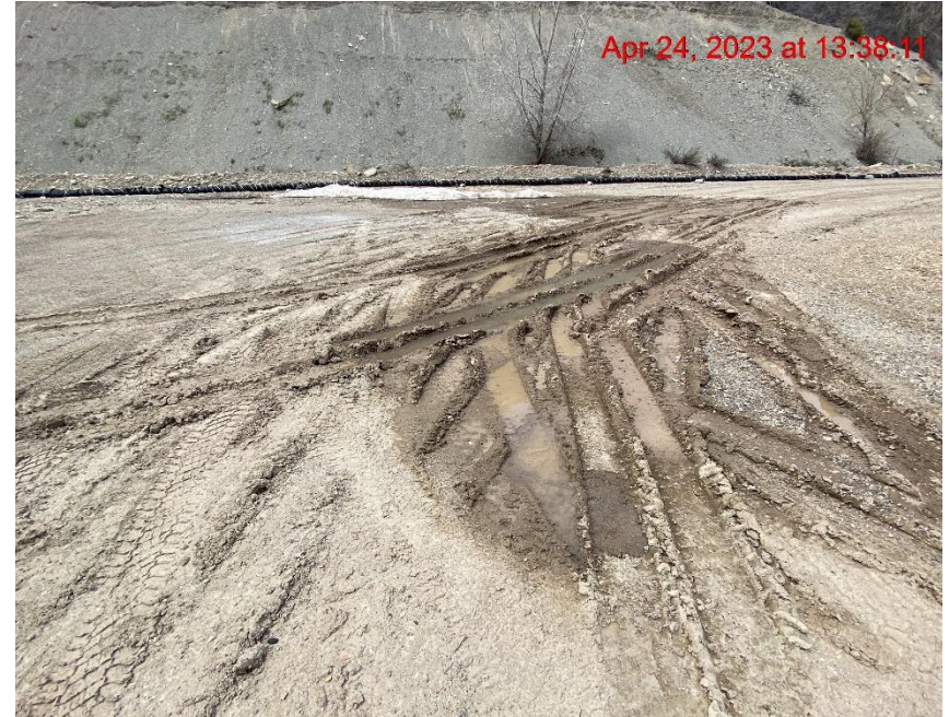
Lack of Stabilization – Photo #02502
