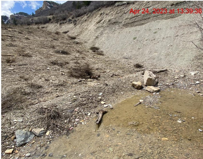
Slope Erosion onto Location – Photo #02506
