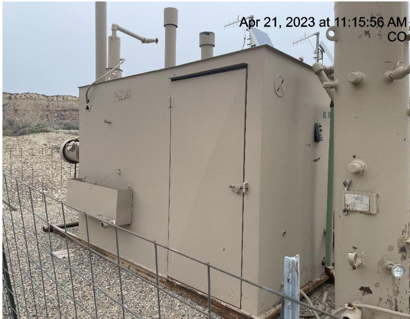
Photo # 6031 Meter calibration info not conspicuously posted
