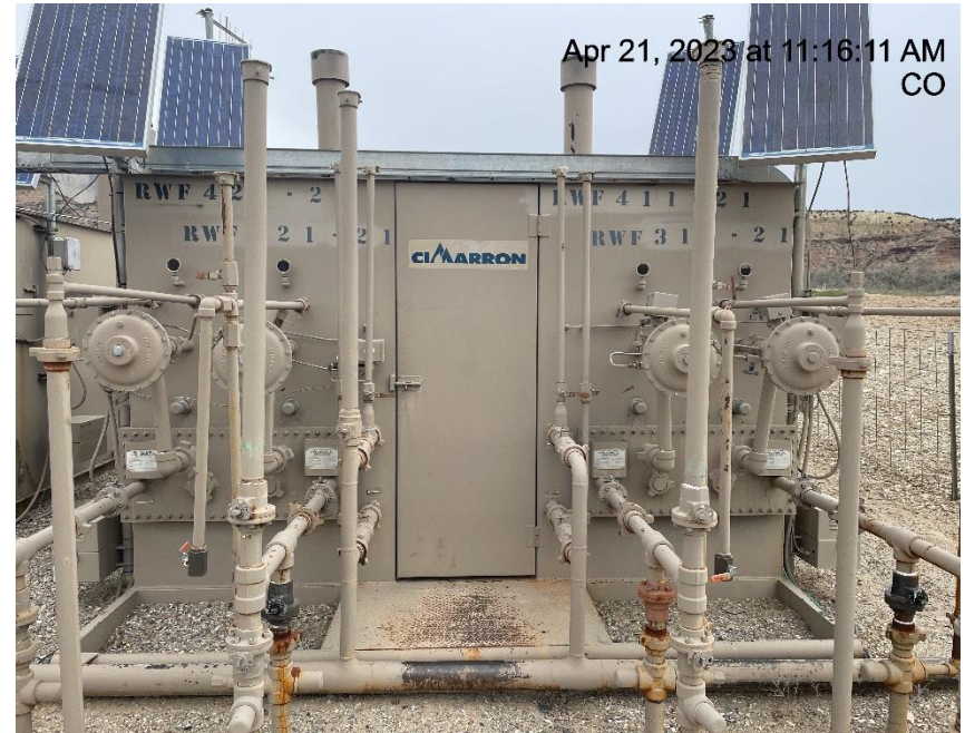
Photo # 6032 Meter calibration info not conspicuously posted
