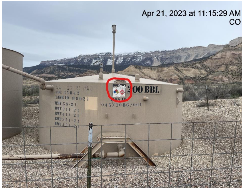
Photo # 6029 Tank label damaged & some info is missing
