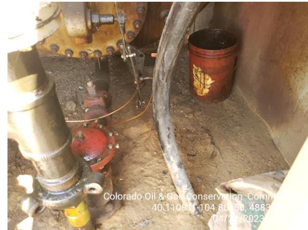
**Photo 9 Stained soil in Heater Treater housing.**
