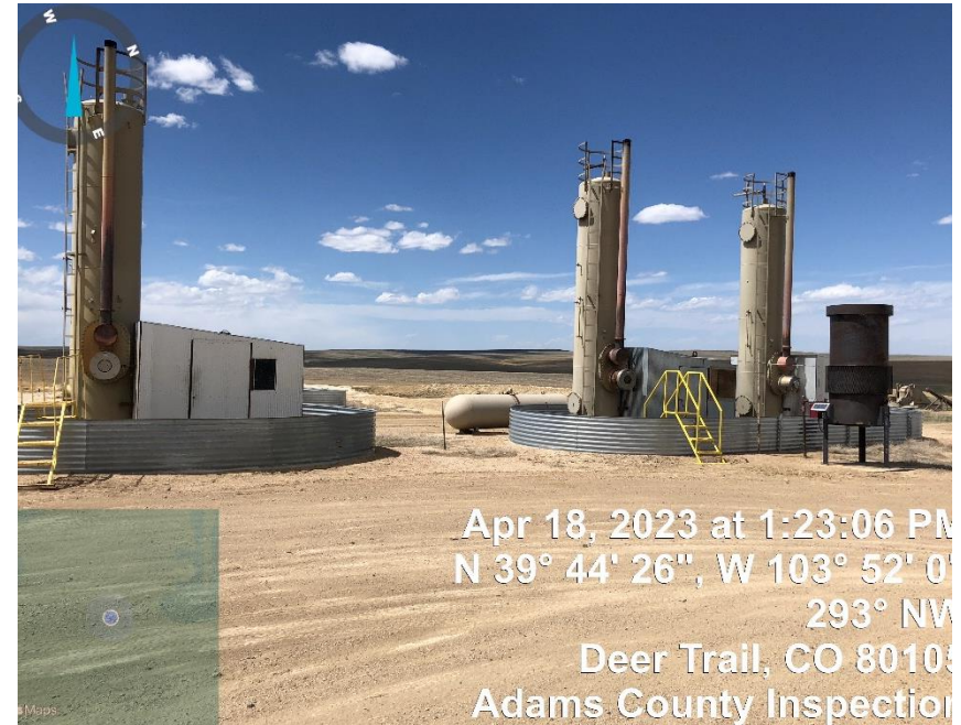
Photo#2 (3) Separators/ECD/Propane Tank
