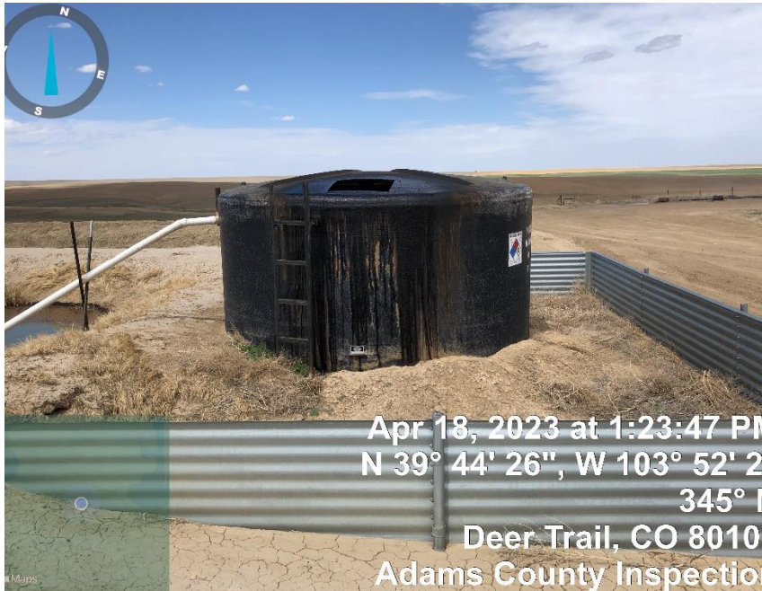
Photo#3 Produced Water Tank/ NO Top over opening
