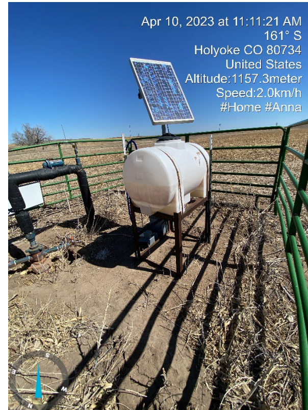
6. Chemical tank without containment.
