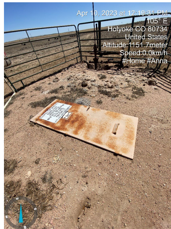
4. Meter shed door laying on the ground
