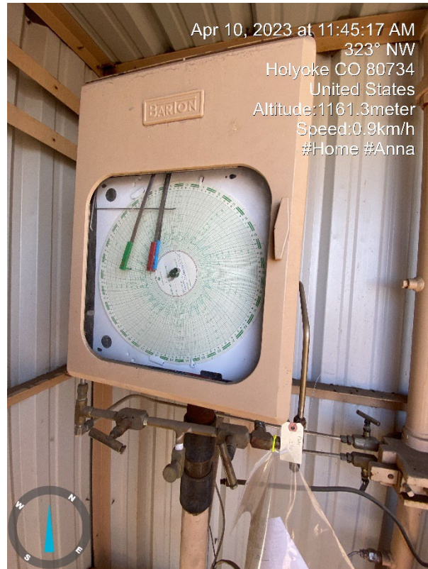
3. Meter run, Chart last changed on 11/30/2022
