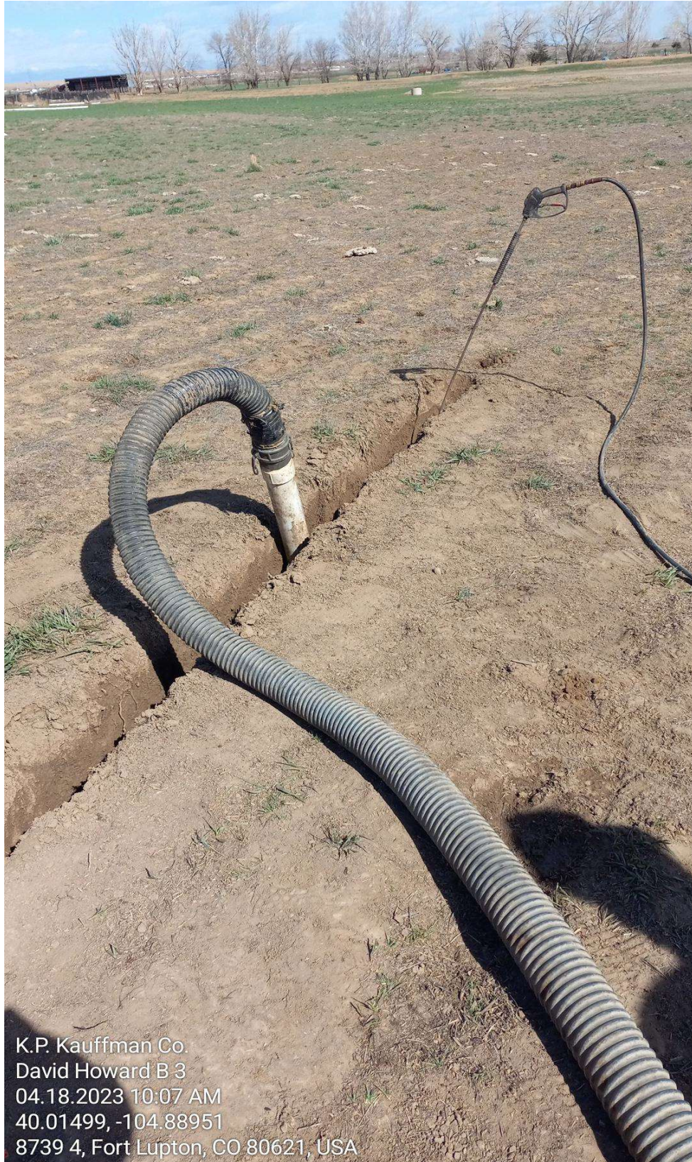
Hydrovac to find landowner water line.
