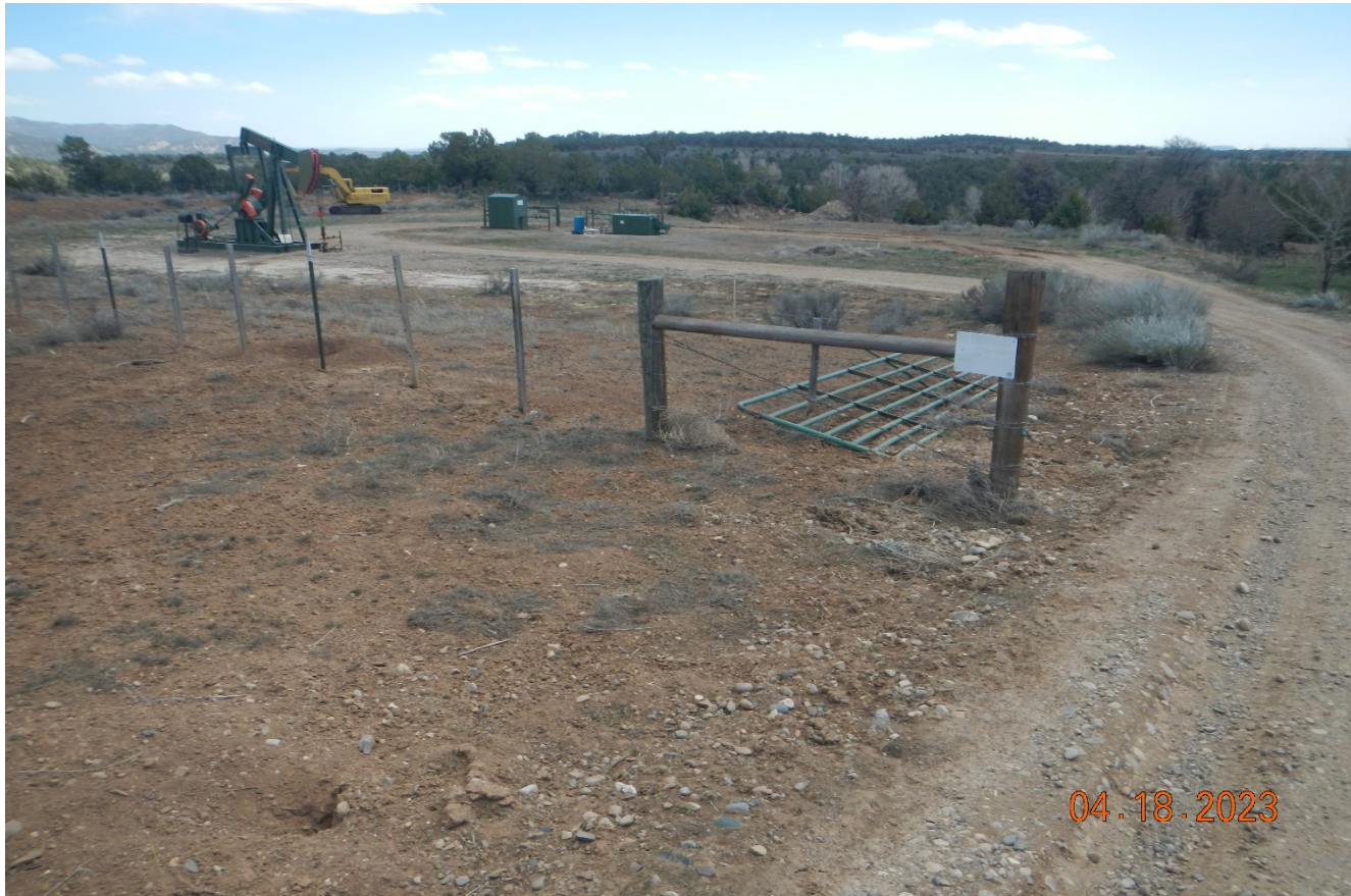
Photo 1. Facing southeast toward the location. The gate has fallen off the hinges and needs to be re hung.
