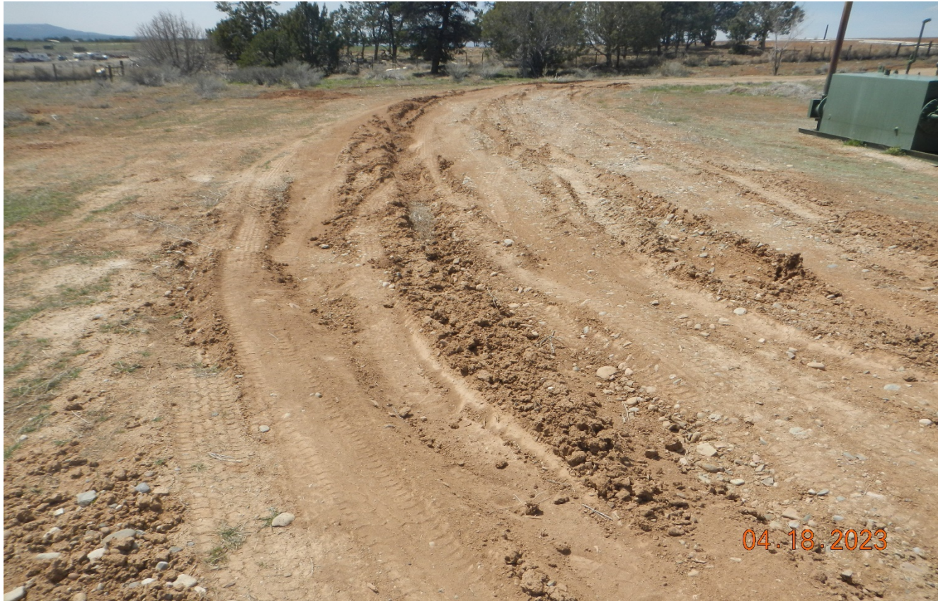
Photo 3. There is vehicle rutting and track at the location that needs to be repaired and stabilized.
