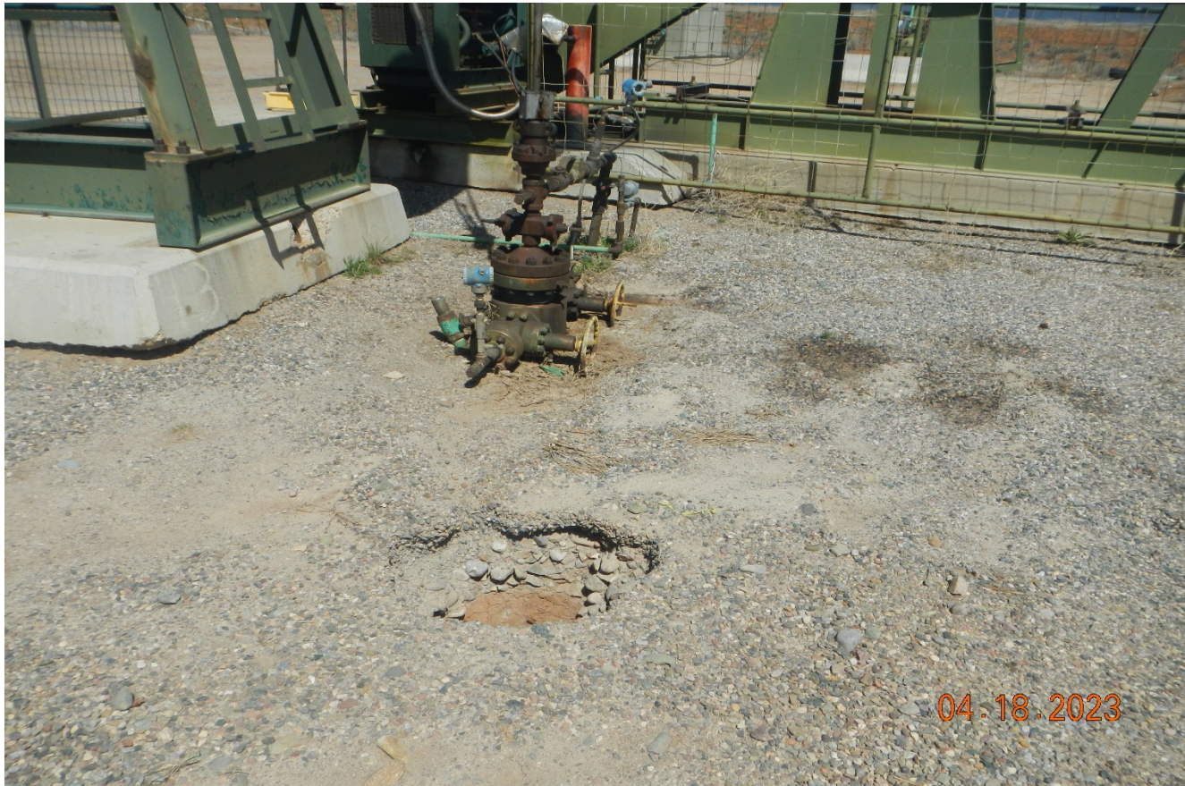
Photo 2. There is a deep hole next to this wellhead that needs to be immediately covered to prevent entry.
