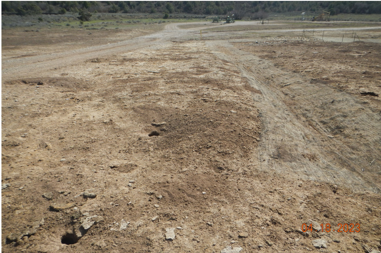
Photo 2. This area along the access road was seeded and hydromulched. The swaled area has straw blanket installed. Seeded areas need to be monitored for vegetation establishment and reseeded if needed.
