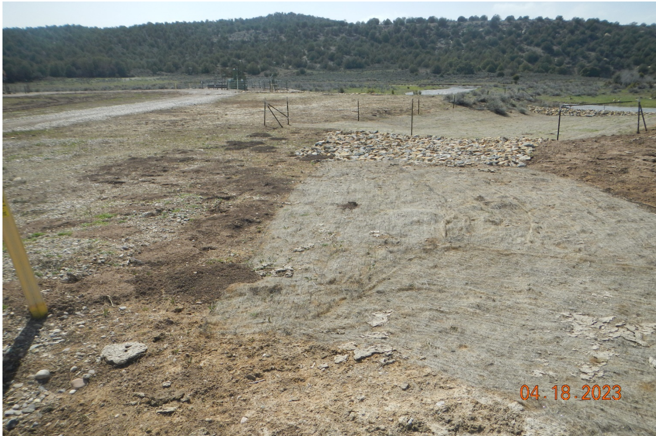
Photo 3. Facing southwest toward the swaled area which has been seeded and stabilized with rip/rap and straw blanket.
