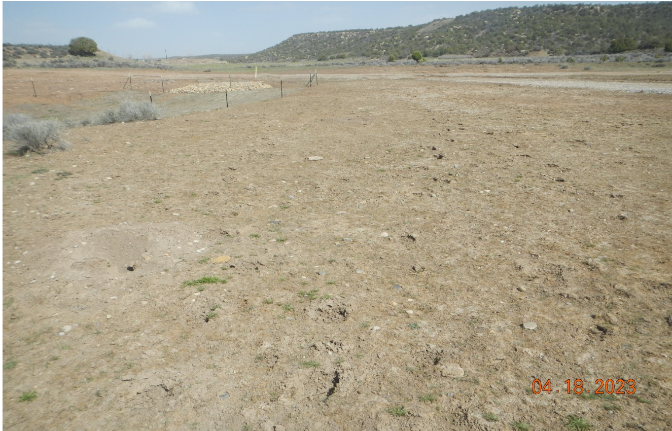
Photo 8. West side of the location facing east. This area was seeded and hydromulched. There was some vegetation germination observed however, seeded areas will need to be monitored to ensure the vegetation establishment progresses.
