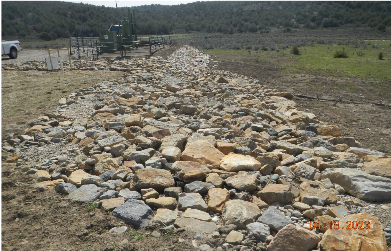
Photo 7. Facing southwest at the west side of the location. This area adjacent to the Florida River has been rock rip/raped. Angular rock was used part of this area which hold together much better than round rock which can become displaced.
