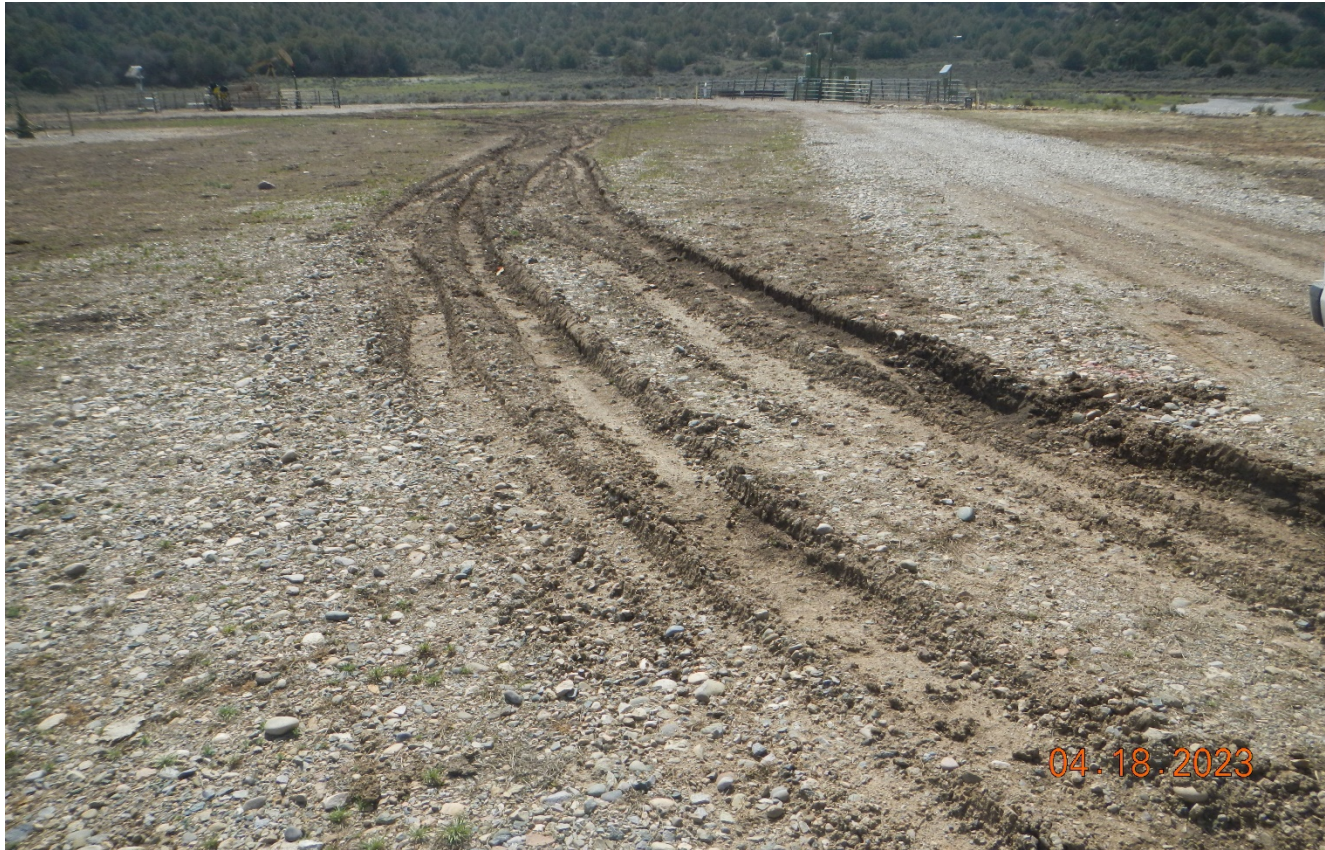
Photo 4. Facing southwest at the location. There is vehicle rutting off the access road and across the location that needs to be repaired and reclaimed
