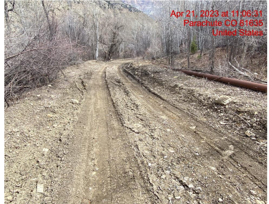
Access Road: Lack of Stabilization/Transportation of Sediment – Photo #02464
