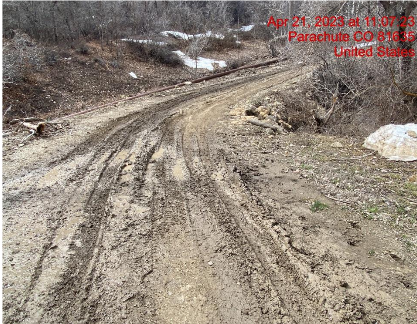
Access Road: Lack of Stabilization/Transportation of Sediment – Photo #02465
