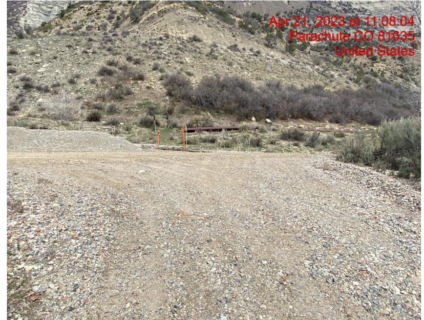
Inadequate Vehicle Tracking BMPs – Photo #02466
