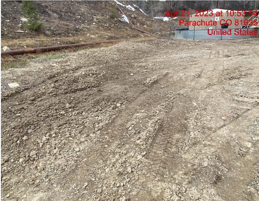
Lack of Stabilization/Transportation of Sediment – Photo #02462
