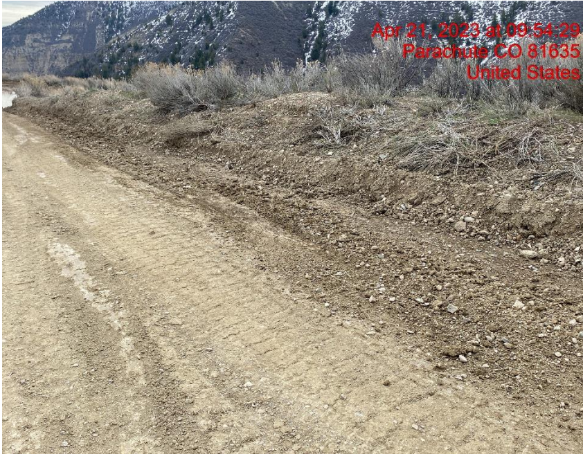
Access Road Degradation/Transport of Sediment – Photo #02432
