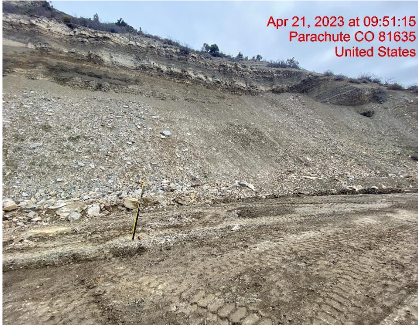
Inadequate Erosion Control – Photo #02425
