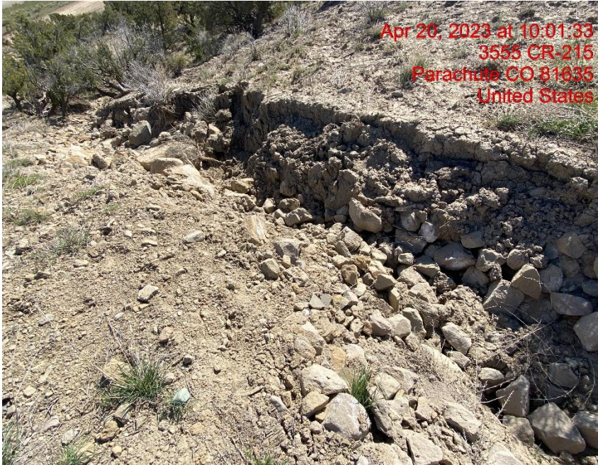
BMP Overrun with Sediment – Photo #02345
