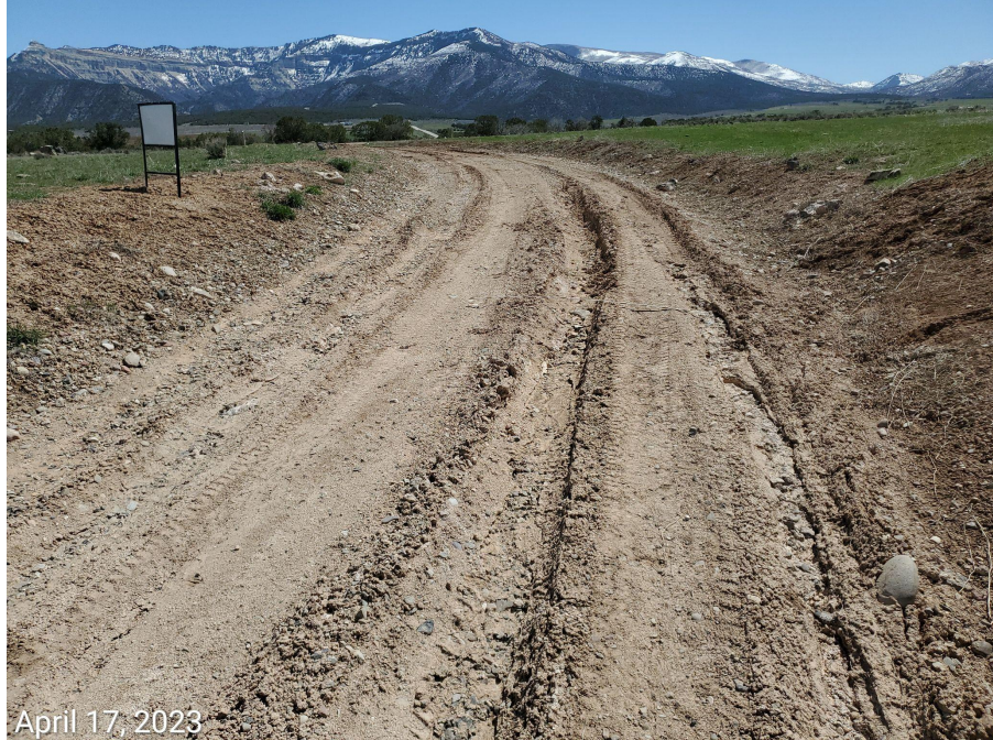
Photo 8: Photo examples showing BMPs at access road are missing or insufficient during wet conditions.
