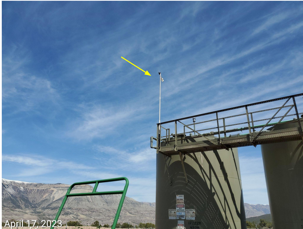
Photo 6: Wind indicator safety equipment not in proper functioning condition.
