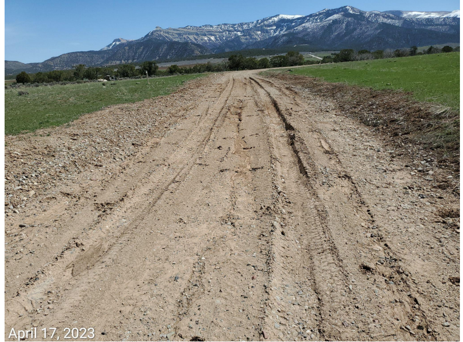
Photo 8: Photo examples showing BMPs at access road are missing or insufficient during wet conditions.
