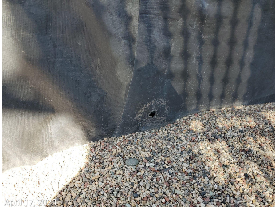
Photo 5: Photos examples showing various holes observed throughout the secondary containment liner.
