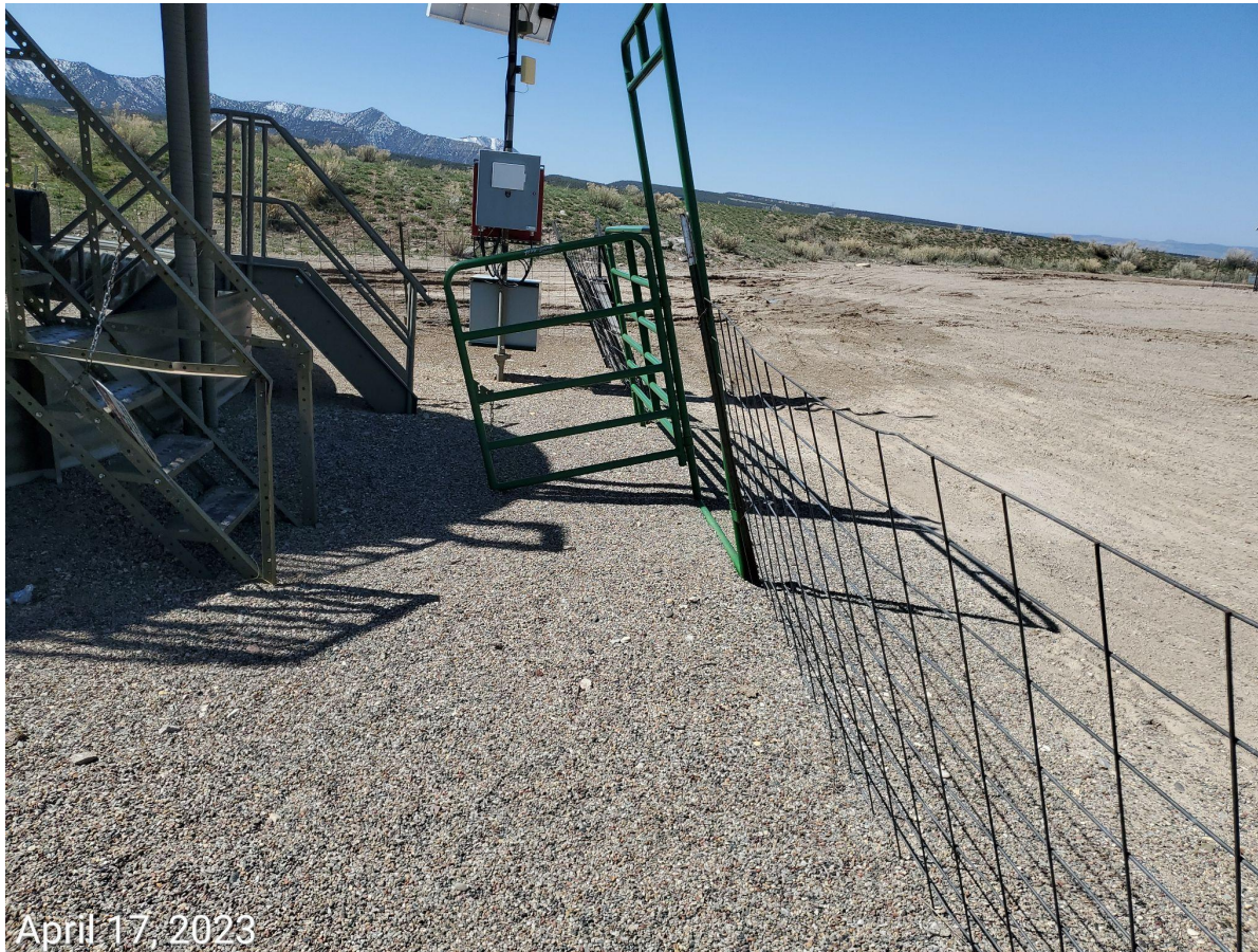
Photo 6: Fence appears to only be supported by the gate- many t-post supports observed to be unanchored.
