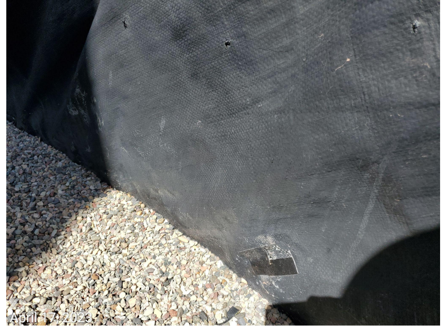
Photo 5: Photos examples showing various holes observed throughout the secondary containment liner.
