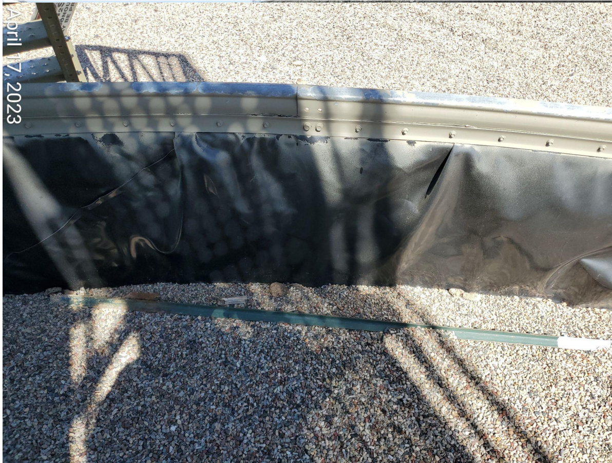
Photo 7: Unused t-post improperly stored within secondary containment of battery.
