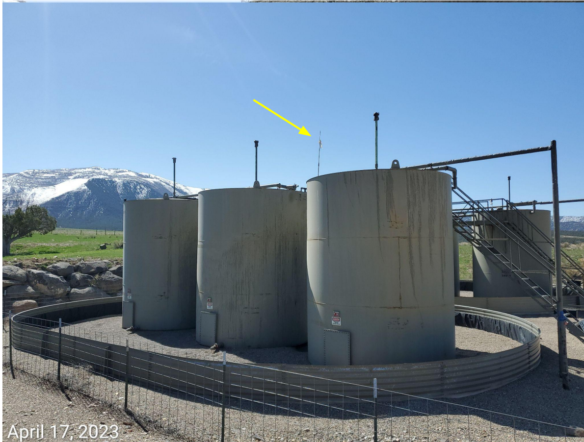
Photo 8: Wind indicator safety equipment not in proper functioning condition.
